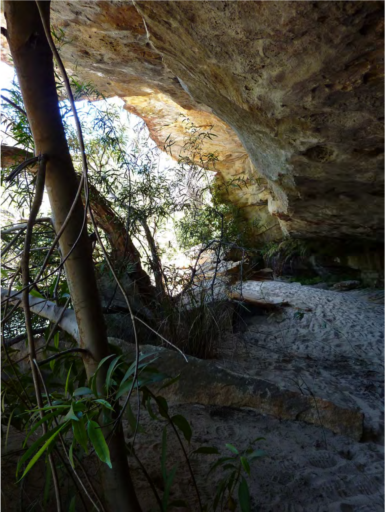
Photo C3-12 Below overhang looking south east
