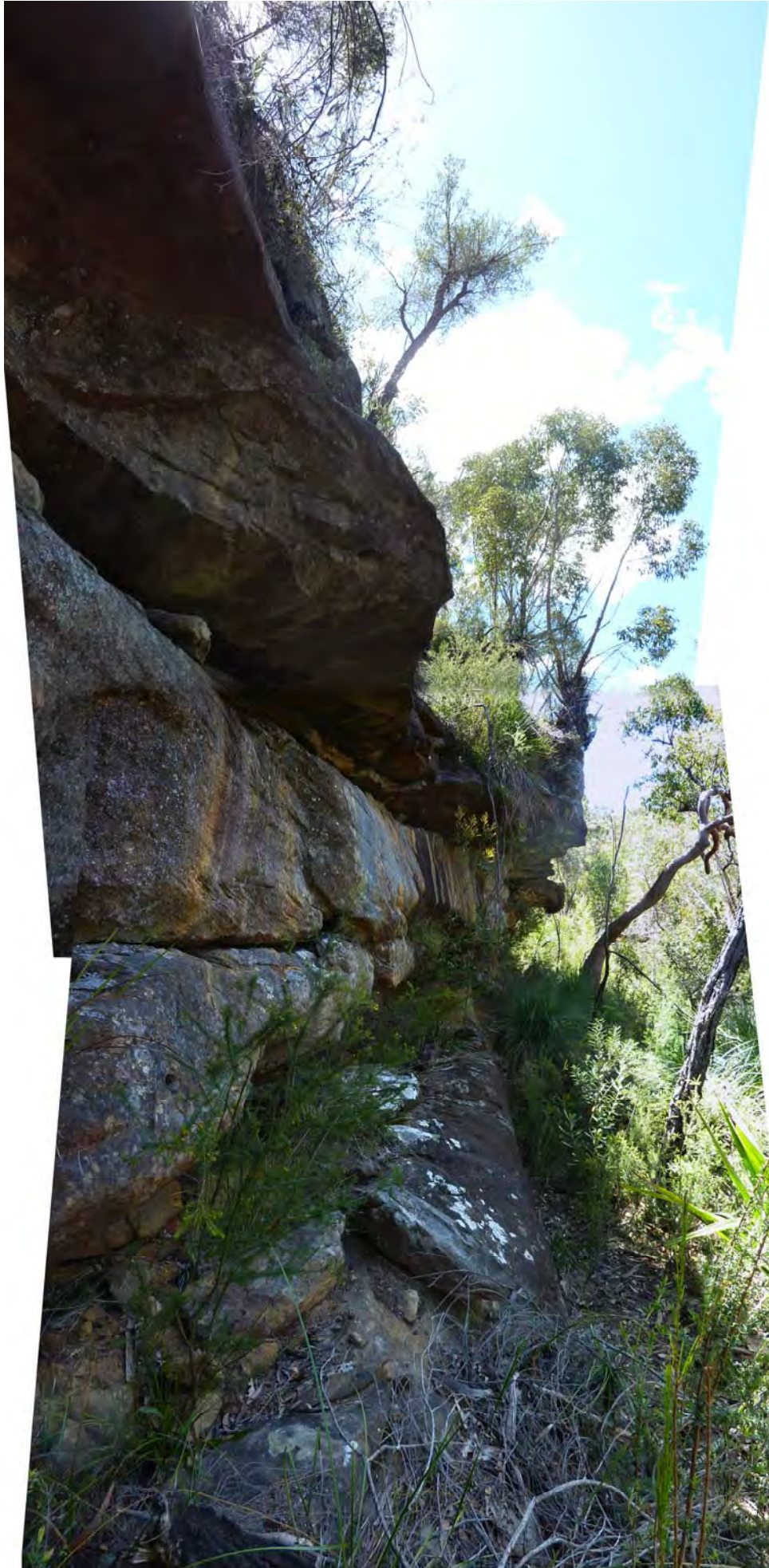
Photo C2-11 Rock ledge between overhangs, ~7.5m high
