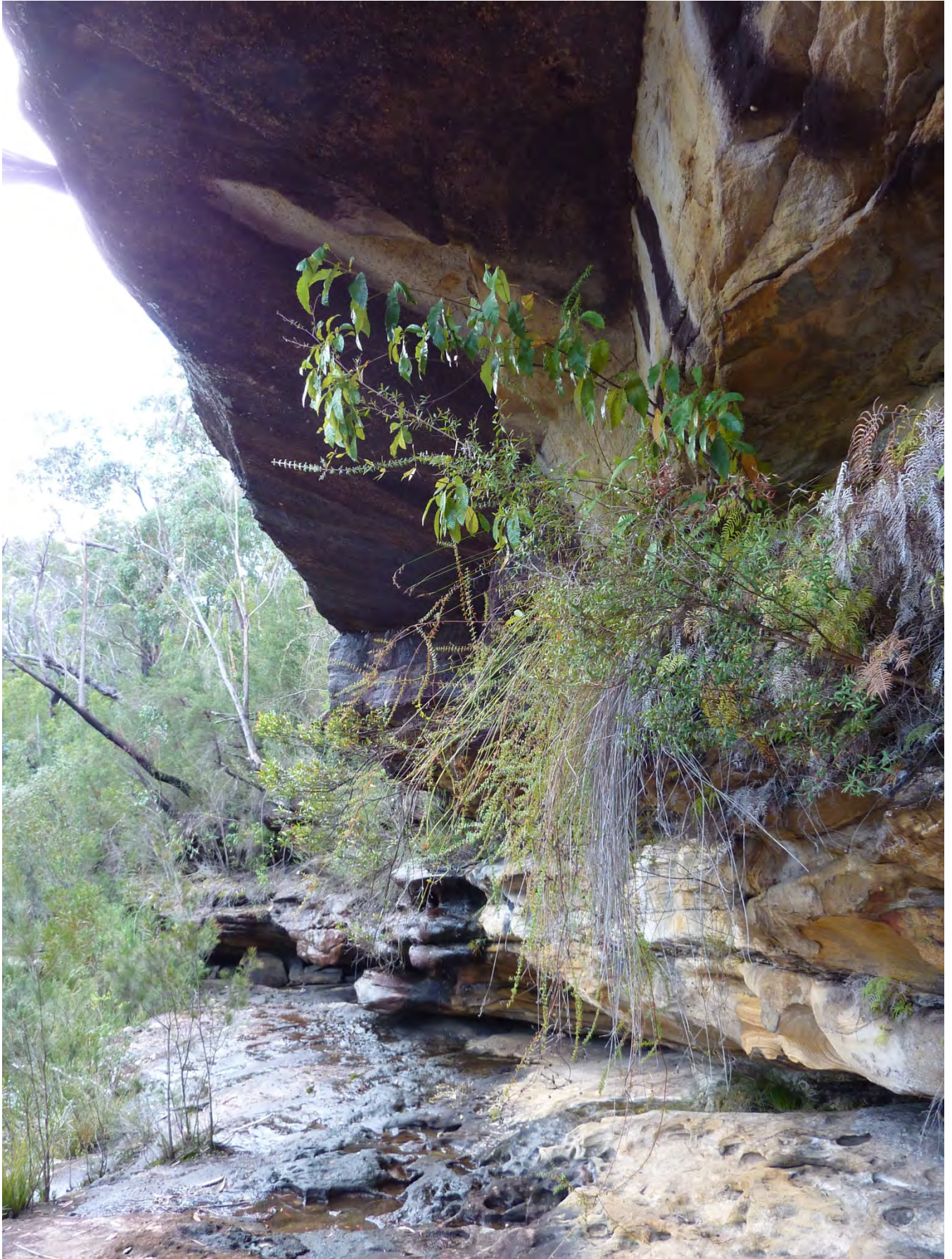
Photo C16-05 Overhang Looking Downstream
