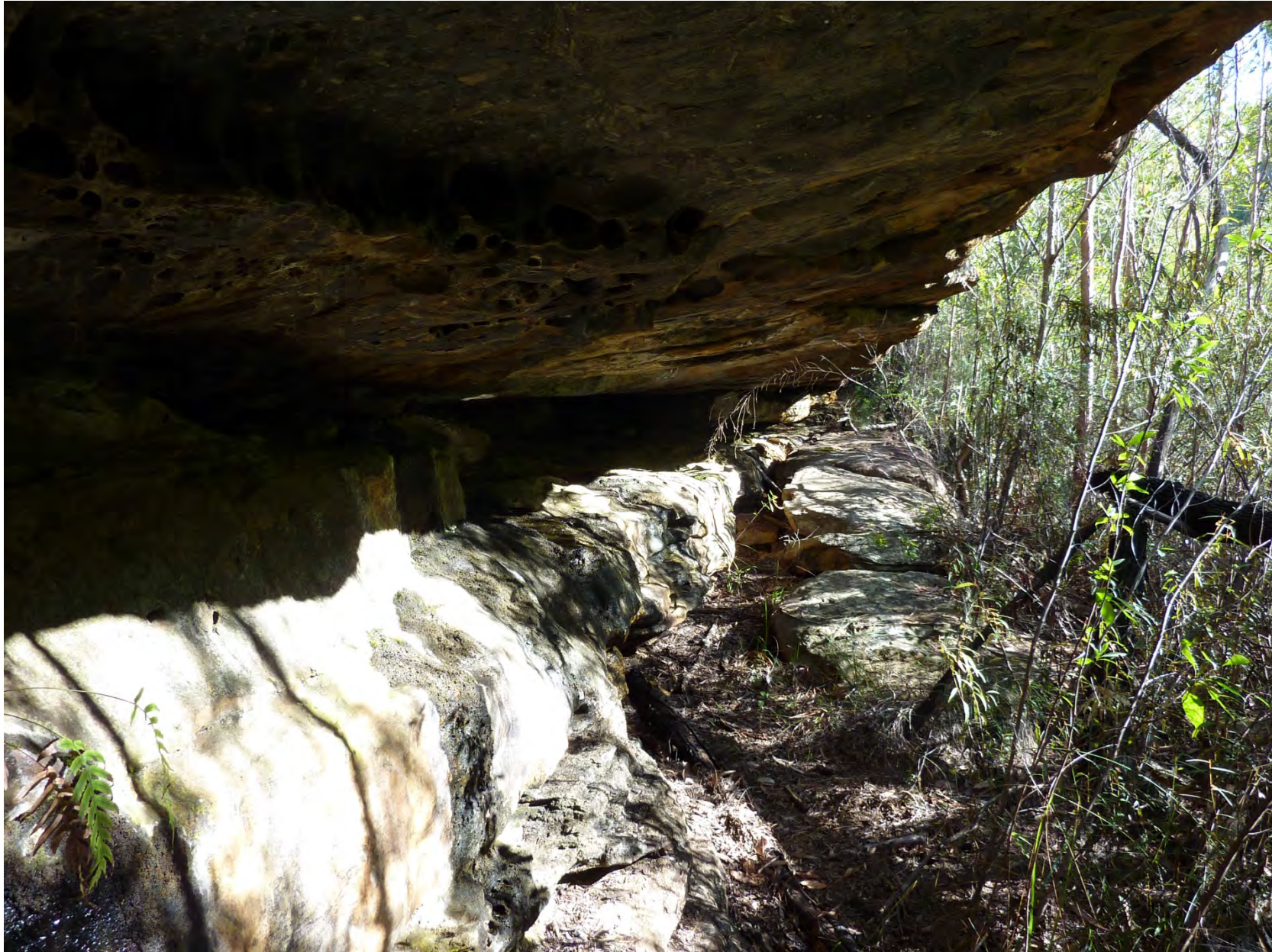
Photo C4-02 Eastern End Looking Upstream
