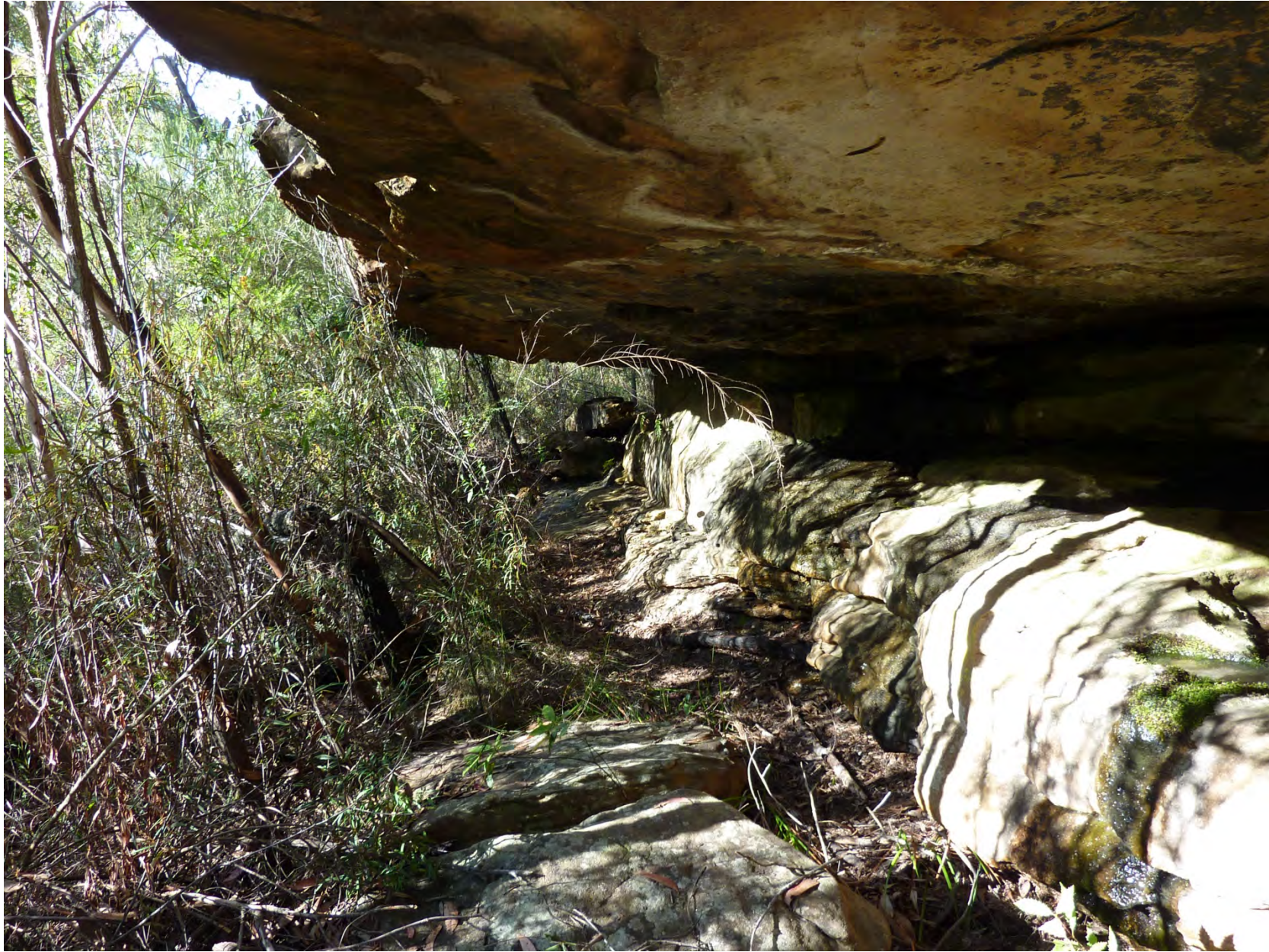
Photo C4-04 Overhang, ~6.5m, Looking Downstream
