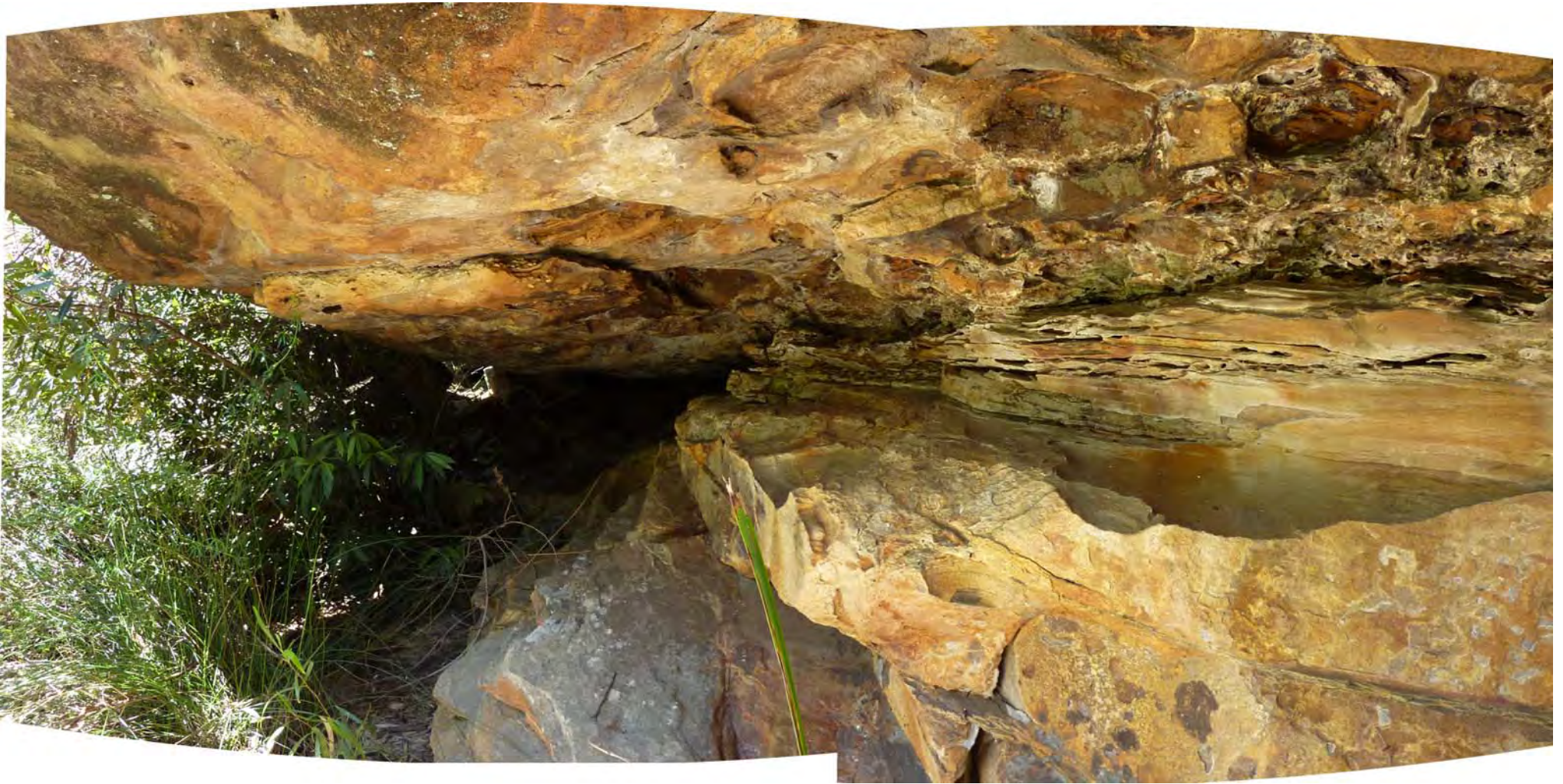
Photo C3-03 Southeast end of overhang, height ~3m to ~5m, depth ~7m
