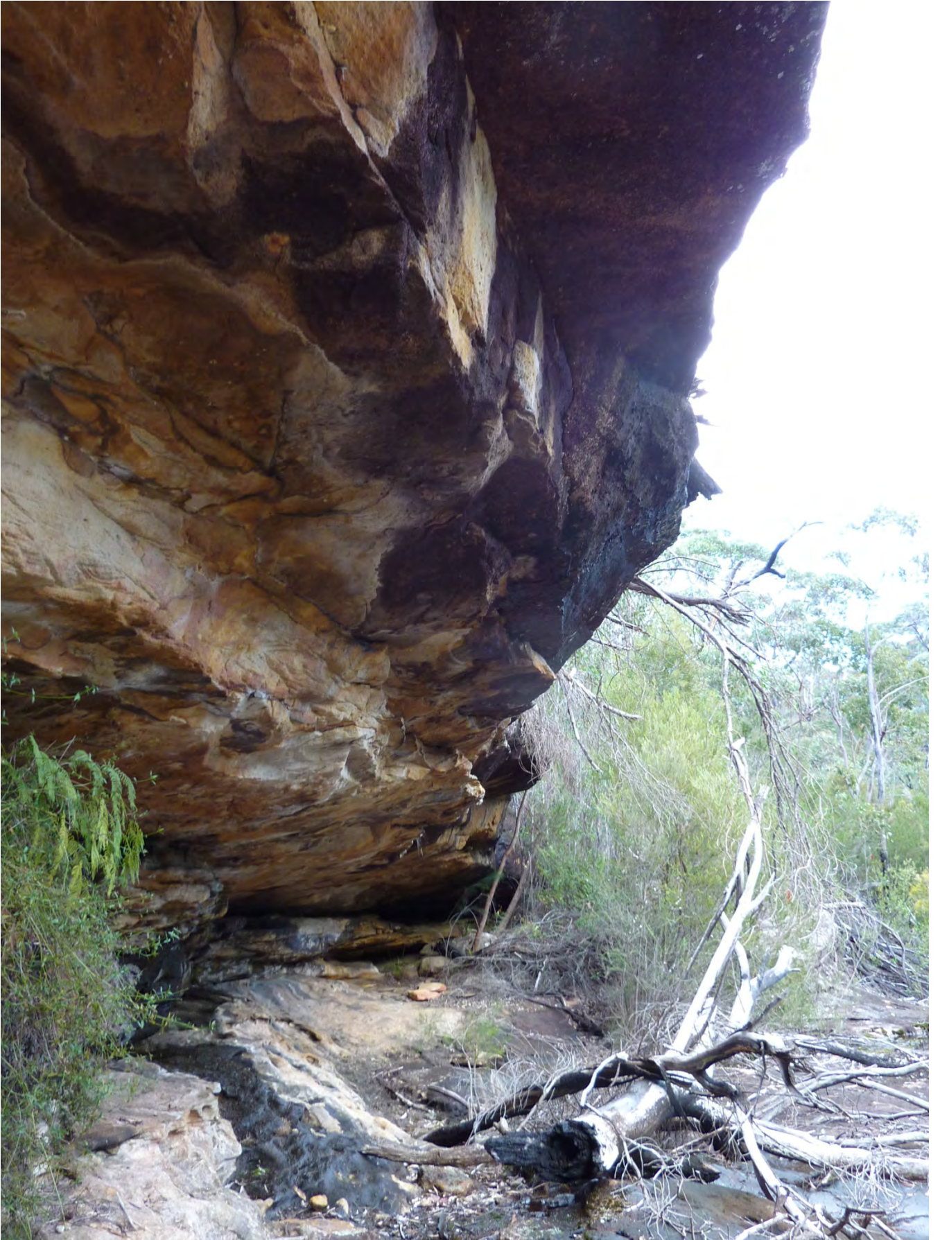
Photo C16-04 Overhang Looking Upstream
