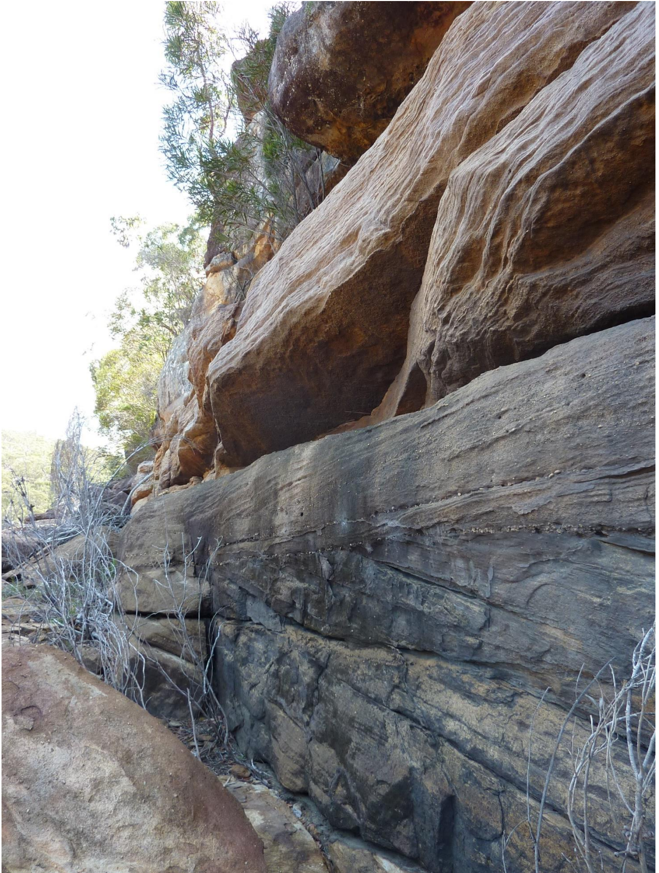
Photo C13-04 South End Looking Downstream
