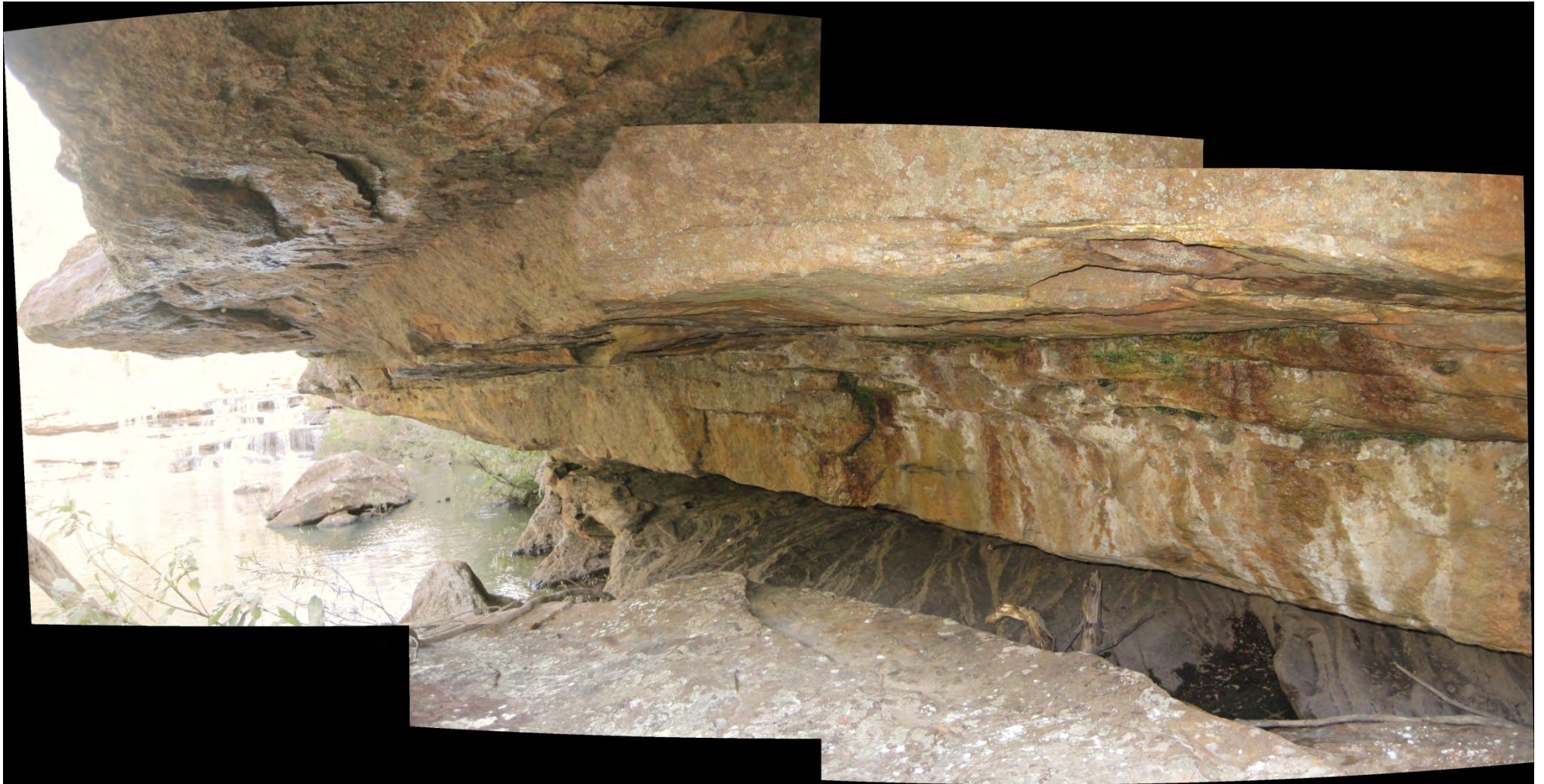
Photo C5-03 Overhang, height ~2.5m, depth ~7m, Looking Upstream
