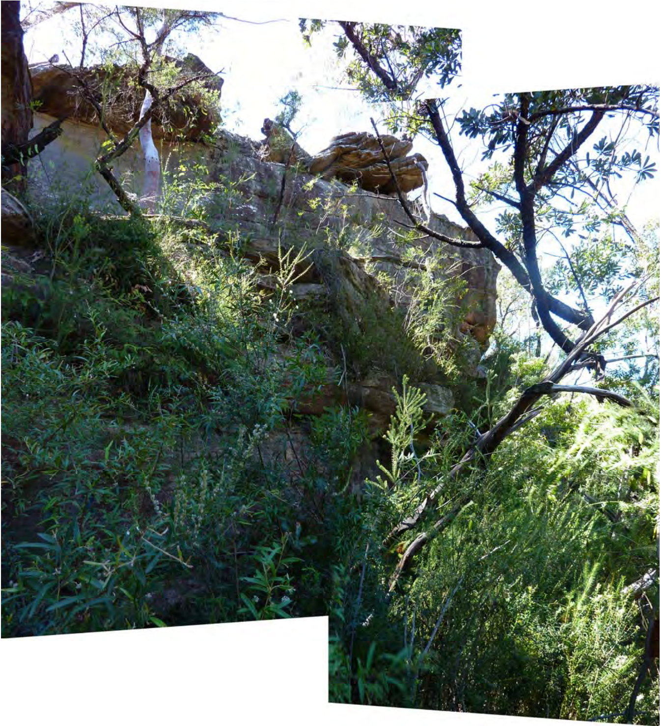
Photo C4-08 Overhang depth ~1m, height ~10m
