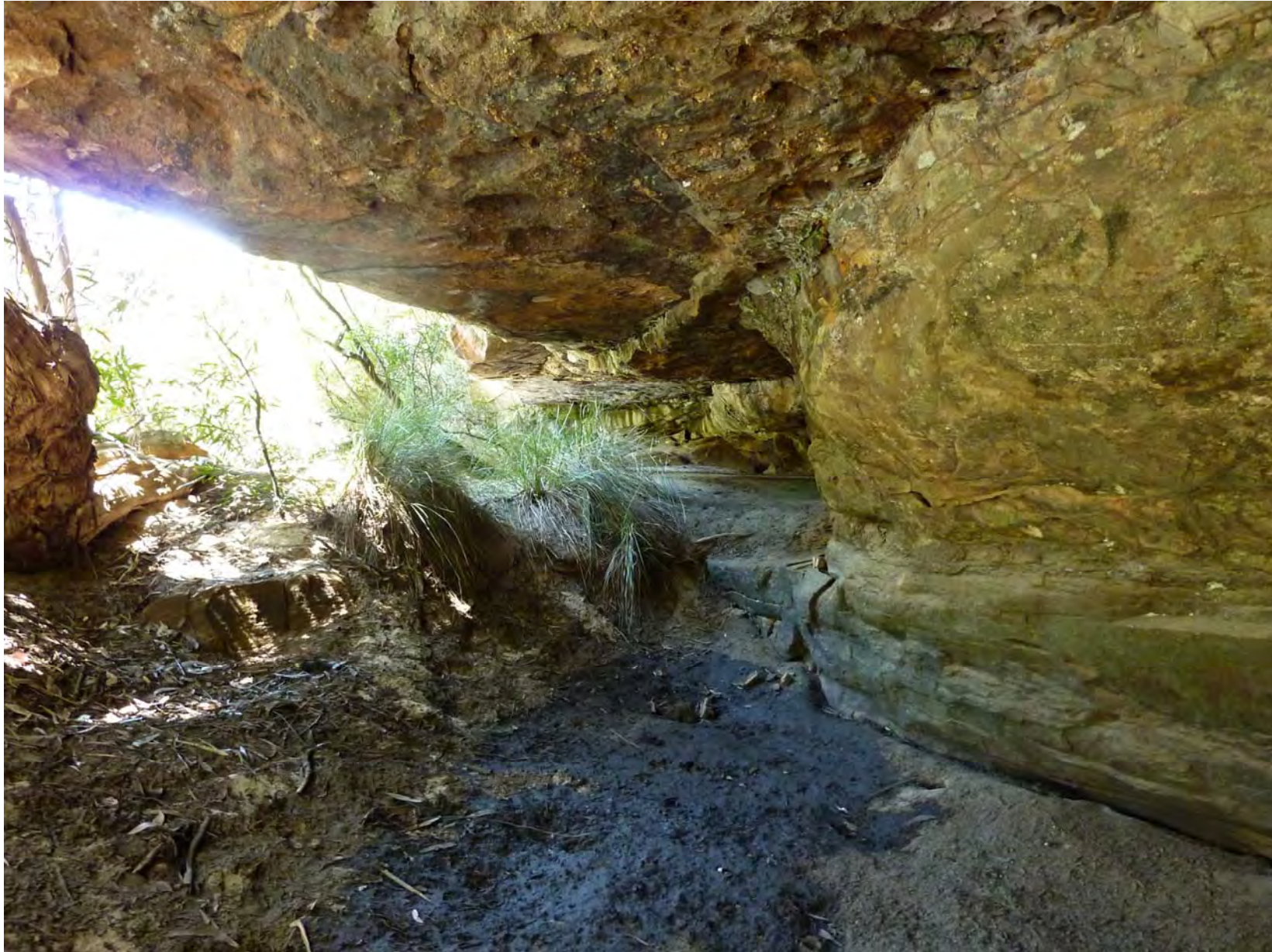
Photo C3-13 Below overhang looking south east
