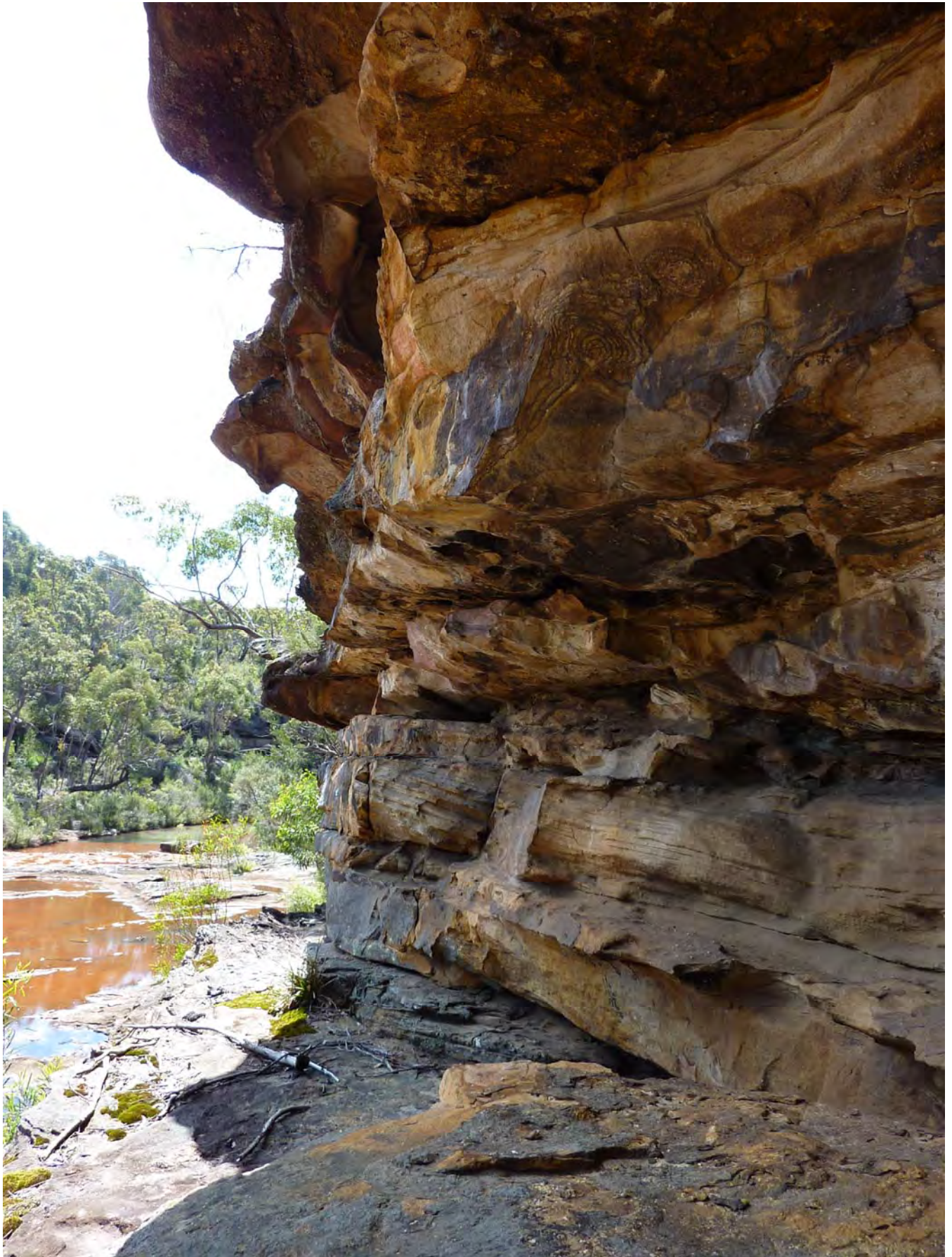
Photo C1-13 Overhang ~5m high, ~3m deep with additional 2m undercut
