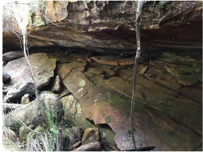
Photo F10 (Upstream 3)
