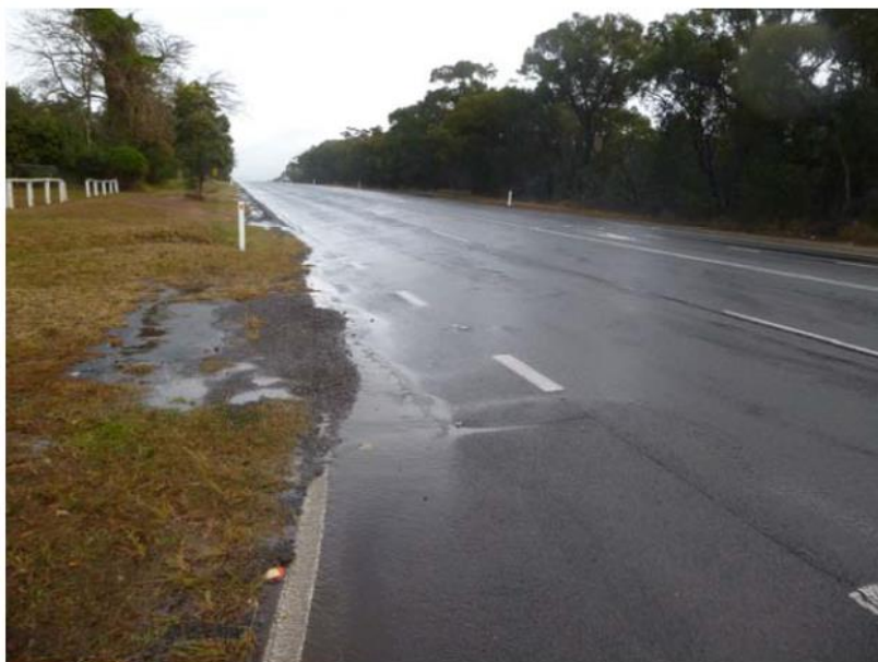
Plate 1 – Old Princes Highway (Source: MSEC, 2016)
