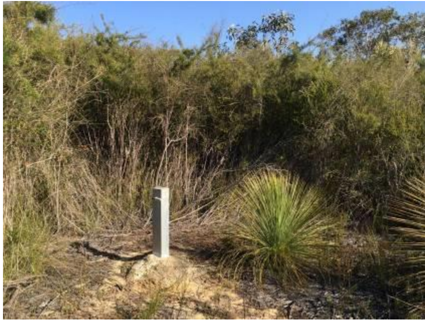
Photo of a typical groundwater bore installation within a swamp. Note vegetation re-establishing within the cleared area following construction.
