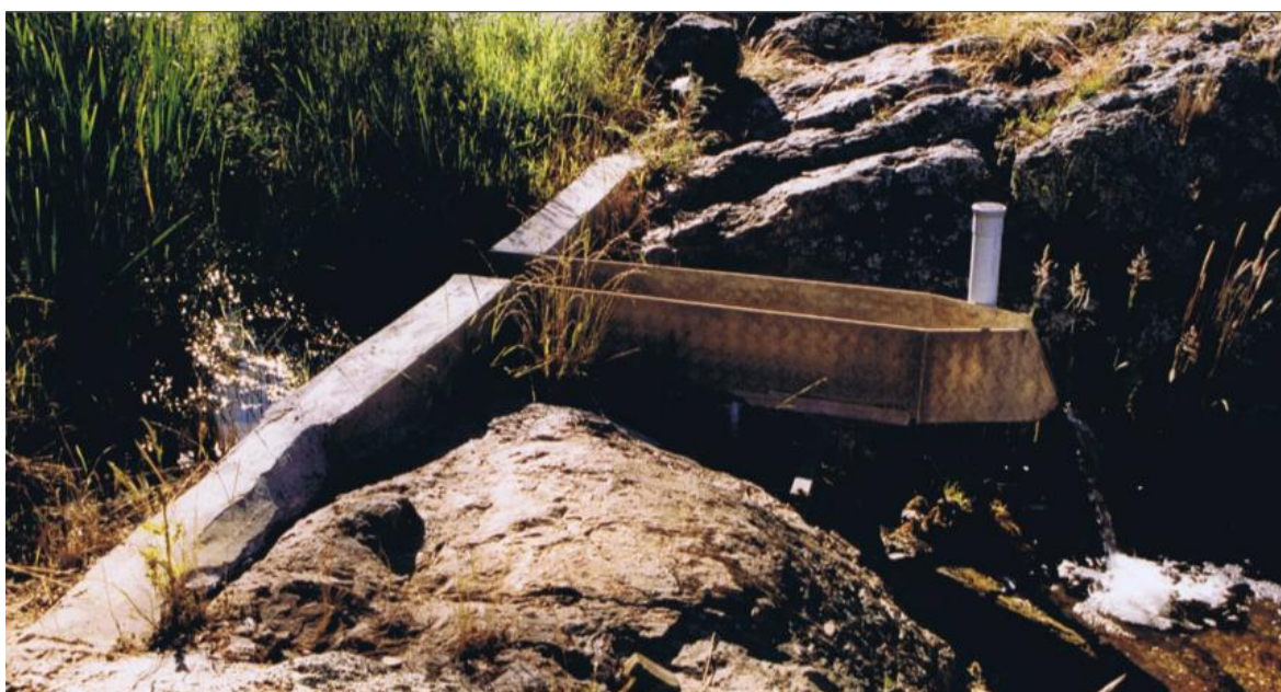
Plate 3 Typical H Flume Installation
