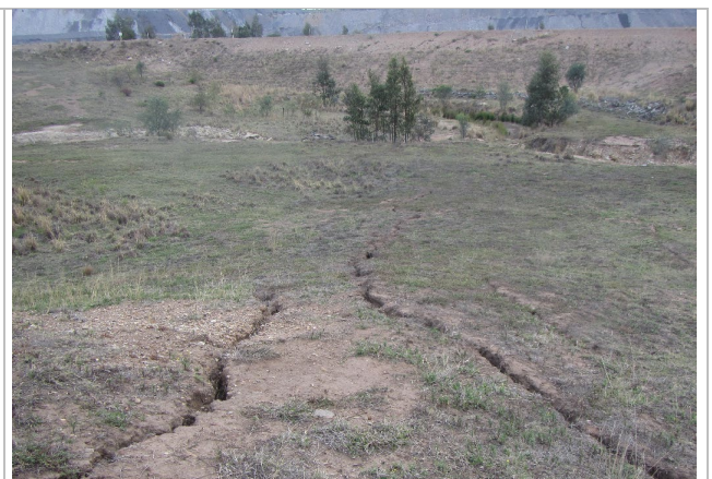
Compression buckle cracks at 1 to 2 m spacing through erodible soil near Div7 over LW 13/14 (2019)
