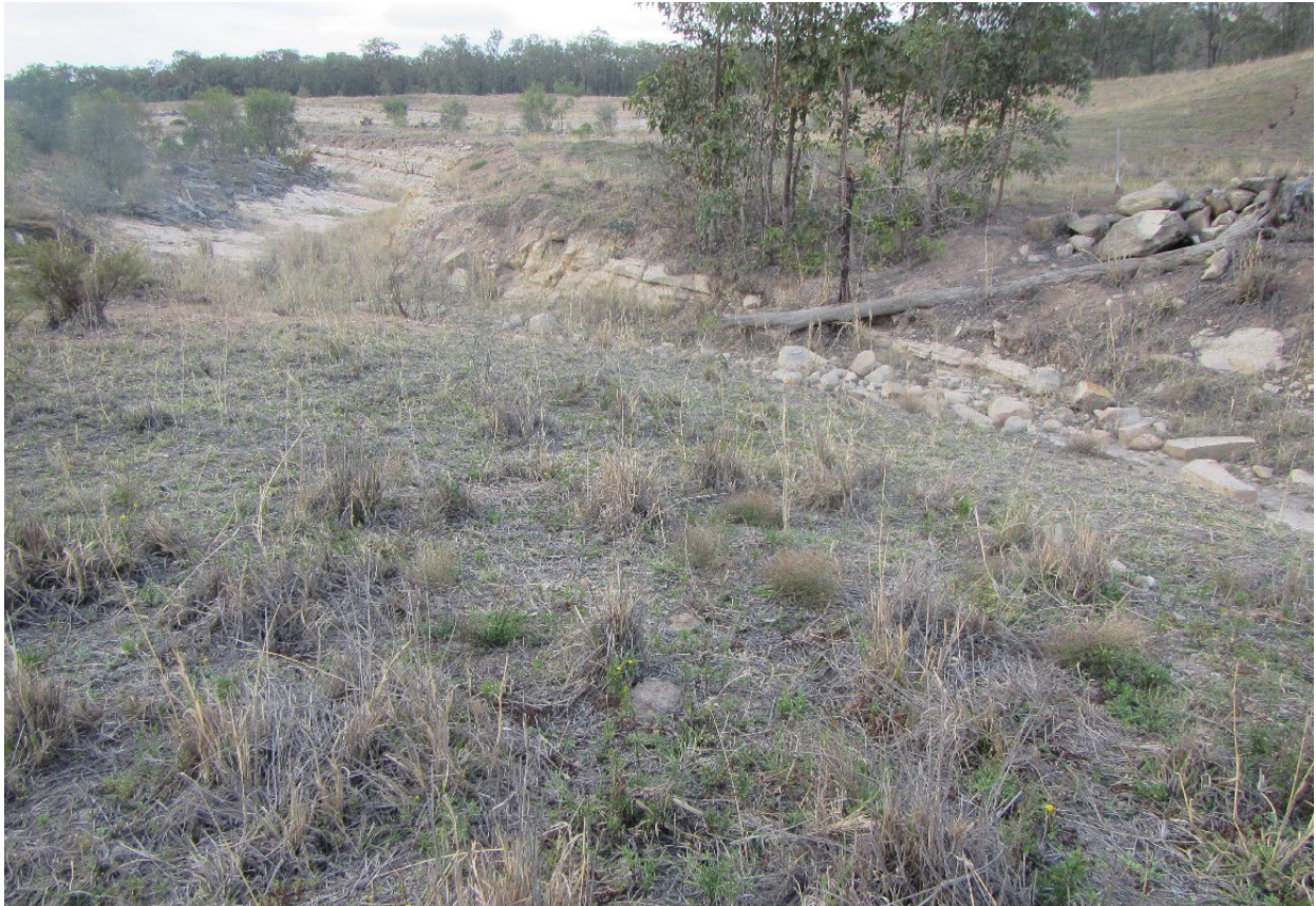
Figure 2-3. Steep, bedrock-controlled transition zone from Stage 2 to Stage 3 showing the subsided drop into LW12/15 (2019)
