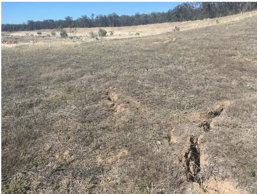
Plate 27: Subsidence cracks near rehabilitation monitoring site 28R
