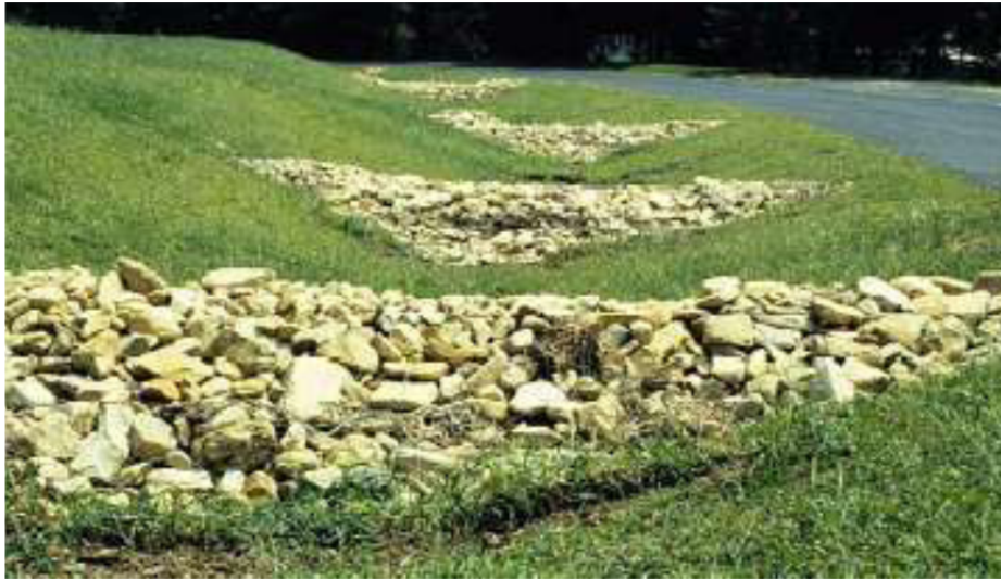
Figure 7: Example of Check Dams
