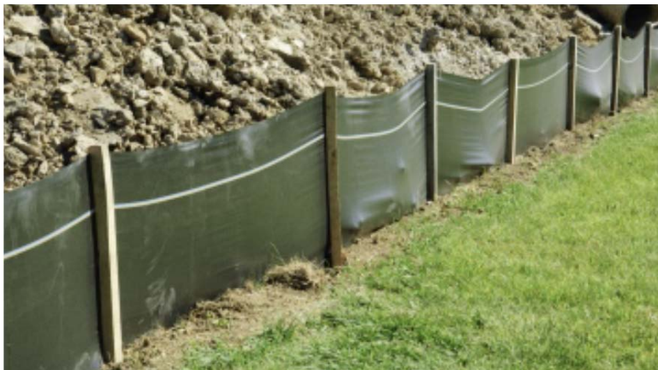
Figure 6: Example of Sediment Fencing
