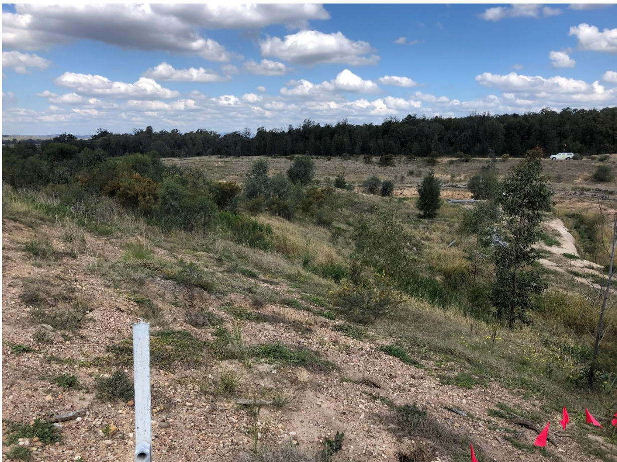
Photograph 20: North Wambo Creek Diversion during 2020 at site 25R showing grasses with native shrubs and some bare soil
