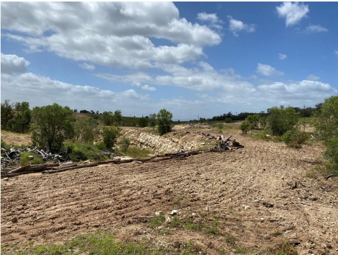
Photograph 22: Example of active soil remediation work in the North Wambo Creek Diversion area in 2020
