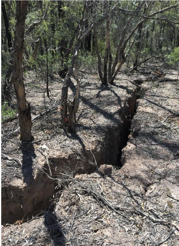
Photograph 39: Large subsidence cracks near flora monitoring site V11-B1 (in 2019)
