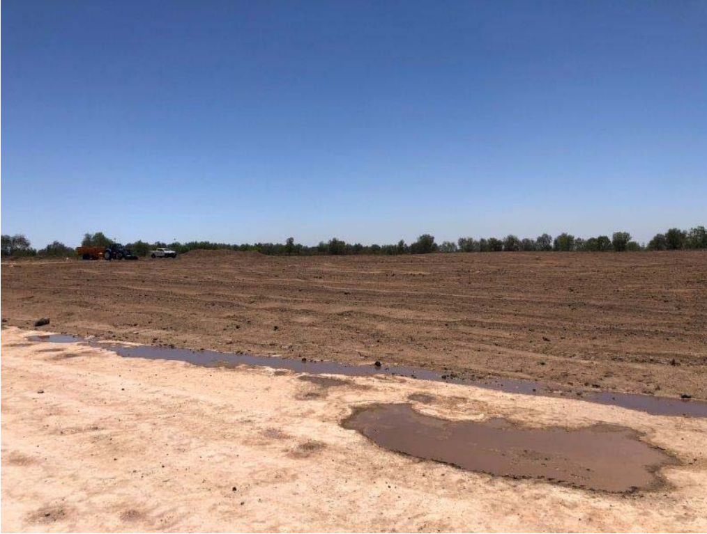
Photograph 7 Preparation works for mine rehabilitation
