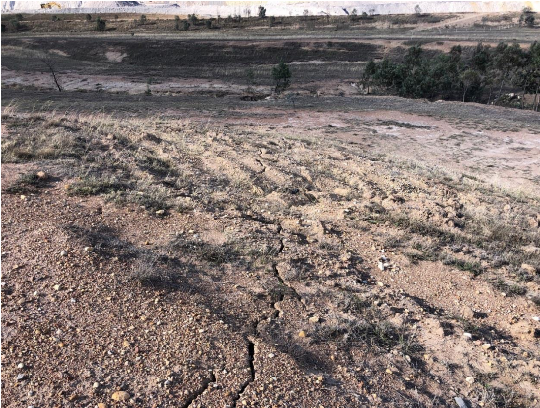
Plate 28. Subsidence cracks, erosion and bare soil along the North Wambo Creek Diversion near site 23R
