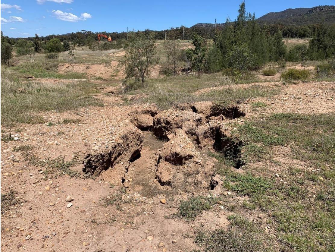
Photograph 18: Gully erosion within the North Wambo Creek Diversion (near site 23R) in 2021
