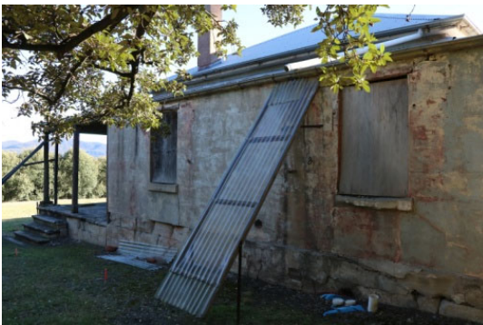
Windows east wall
