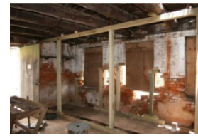
Propped lower floor
