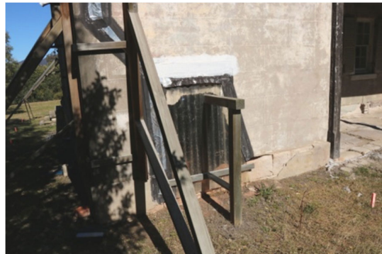
East wall, north corner (props and closures)
