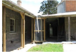
Junction with kitchen
