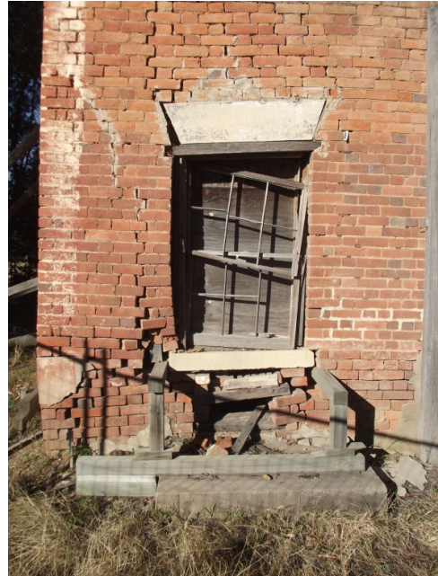
Figure: the north-west corner 2017 Source: EJE 2017
