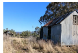
Barn N-E corner
