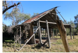
Main shed N-E corner
