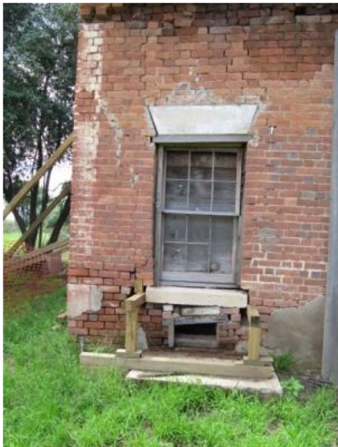
Figure: the north-west corner 2012 Source: GML 2012
