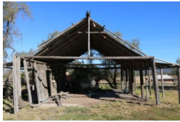
Main shed north
