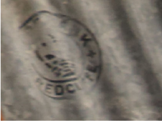
Figure 3.3.8.7: Barn Roof - Redcliffe Crown roofing, imported until 1921. Source: EJE 2017
