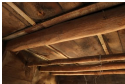
Beams & fine mesh
