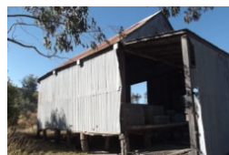
Barn S-W corner
