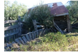
East small shed
