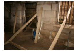
Basement after propping
