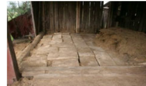
Stone flagging in south end
