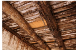
Under upper floor
