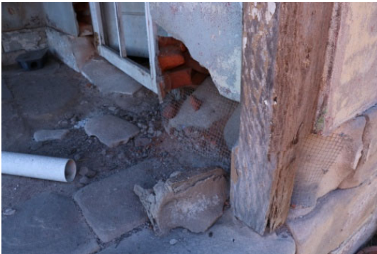
South door, east verandah
