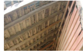
Shingles visible below later roof sheeting
