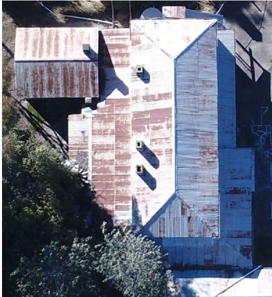
Figure: Kitchen Wing Roofs Source: Peabody Energy 2017
