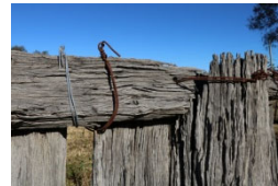
Wire repairs
