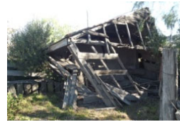
North small shed
