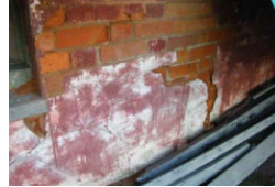
Condition of walls
