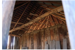
Battens and shingles
