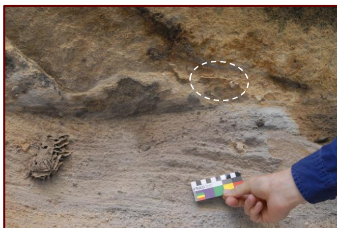
Areas of exfoliation noted in 2020 (DSC_0358)
