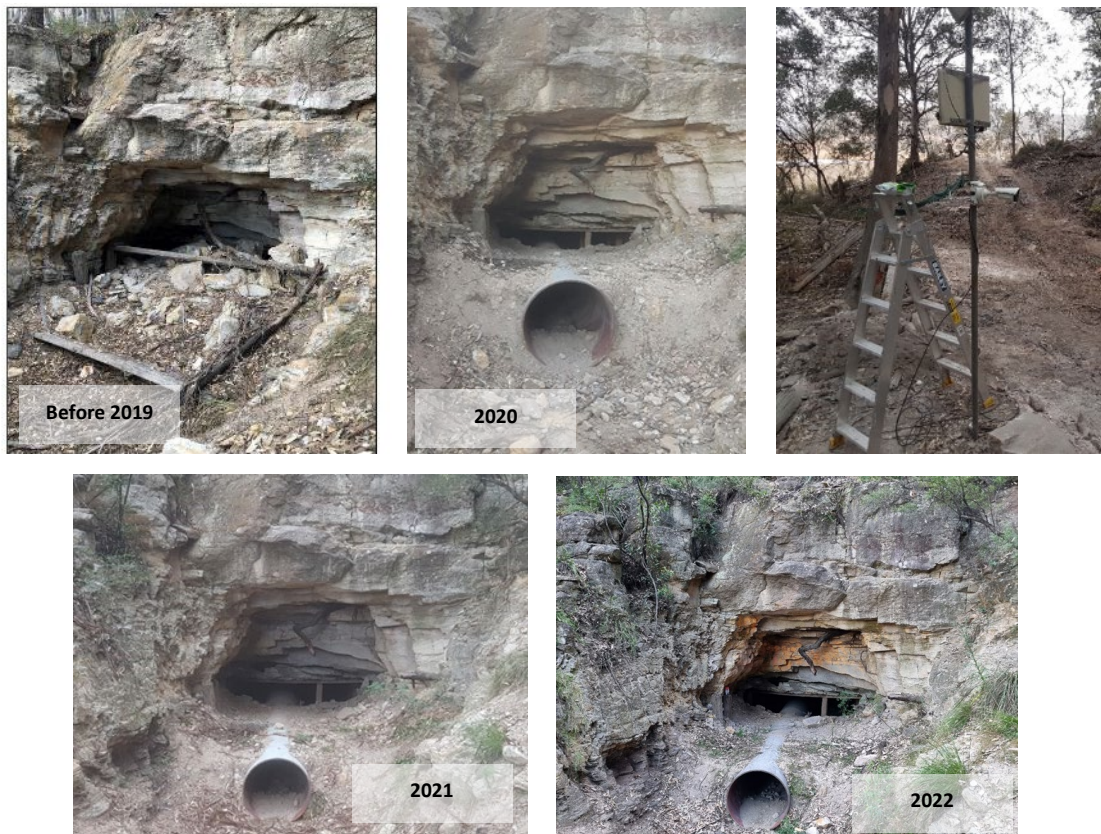
Photo 1 Culvert Support & Bat Detector with Solar Panel setup 20m in front of Adit
