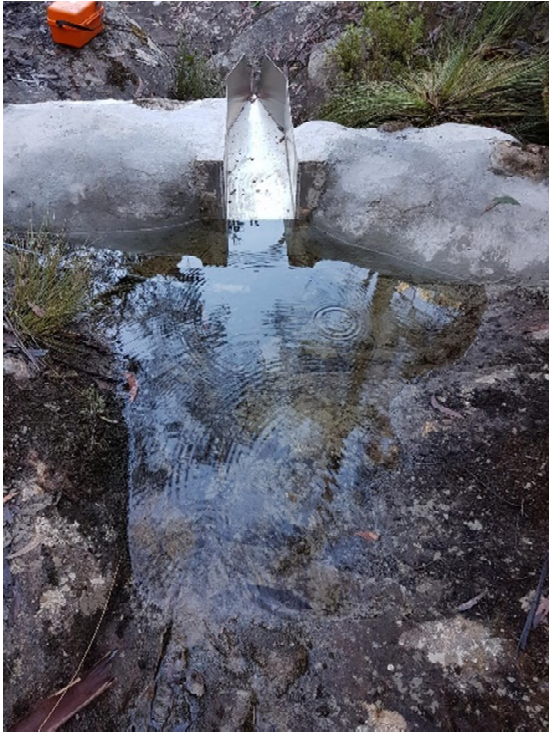
Figure 6.2 Sub-catchment I Flow Gauge (source: Metropolitan Coal)
