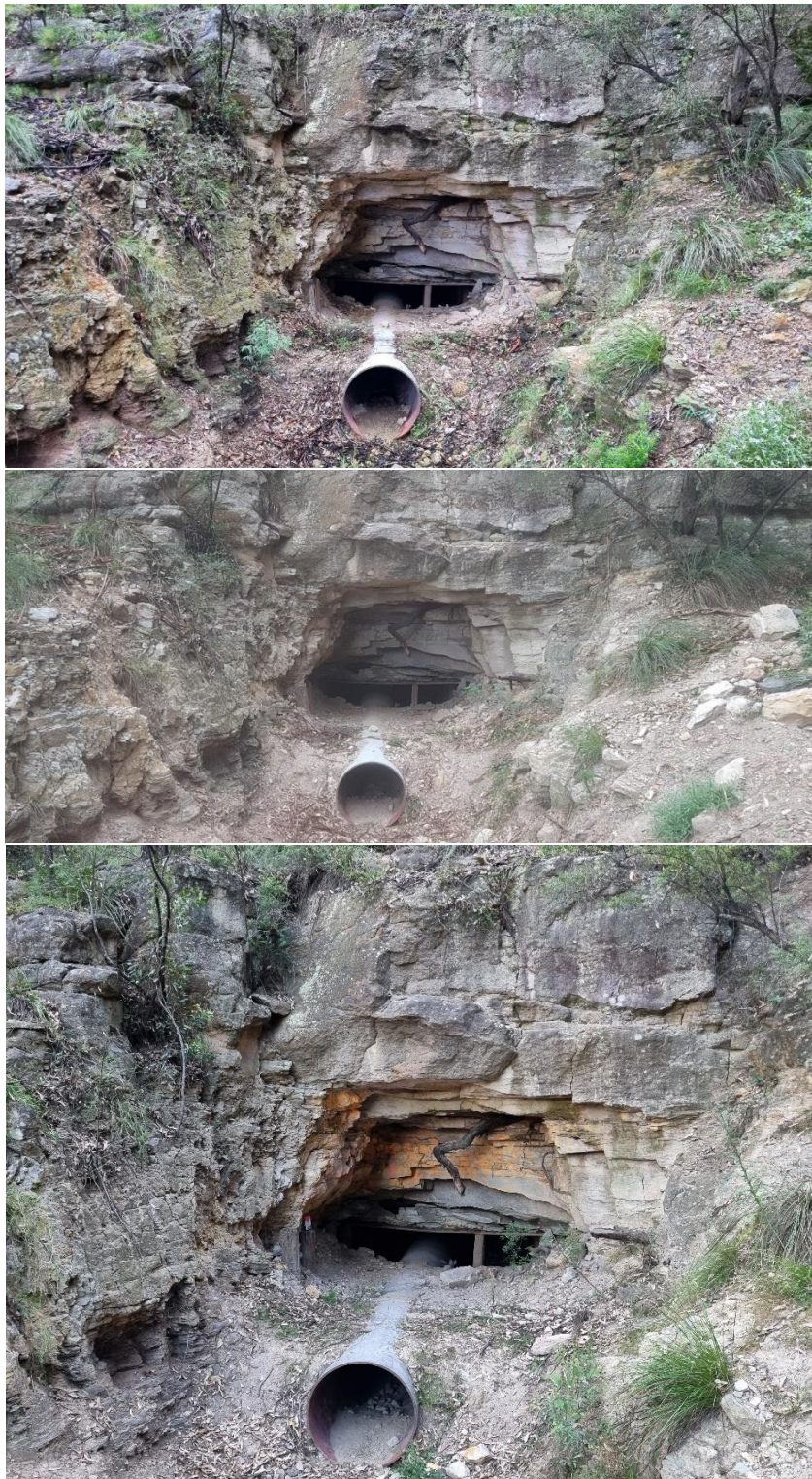
Plate 5-1: Periodic monitoring photo of adit entrance from February 2021 (top), January 2022 (middle) and December 2022 (bottom) showing lack of substantial change
