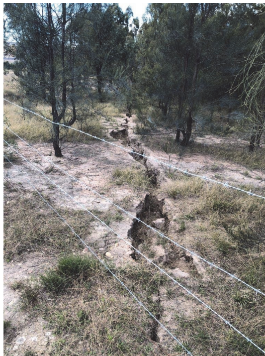
Fig. 4.13 Surface cracking near Dam d07 adjacent to the maingate of WYLW20 (Source: WCPL)
