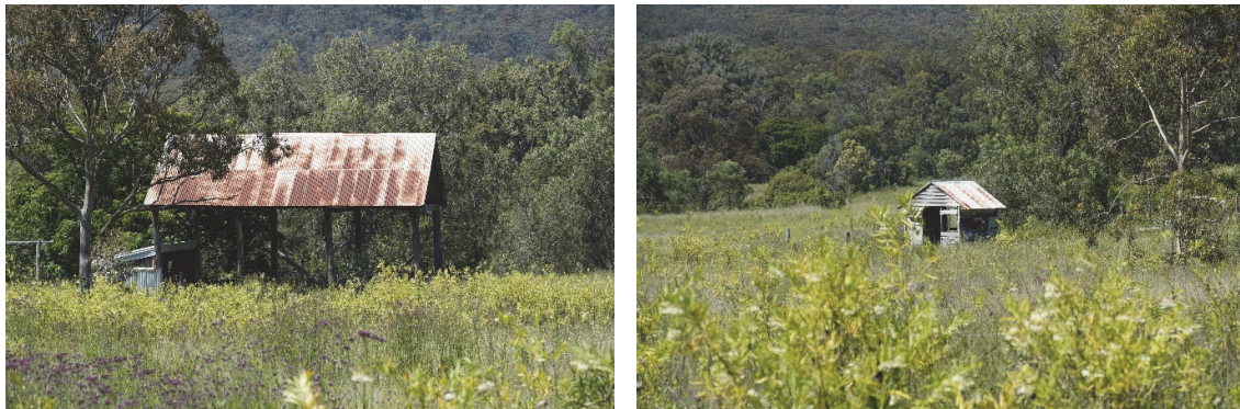
Fig. 6.3 Unused sheds located above the southern end of the proposed WYLW26
