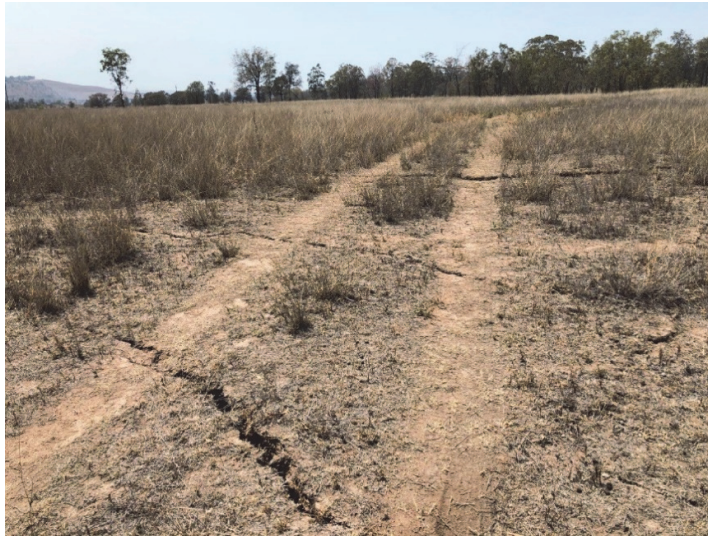
Fig. 4.9 Surface cracking near the finishing end of WYLW18 (Source: WCPL)
