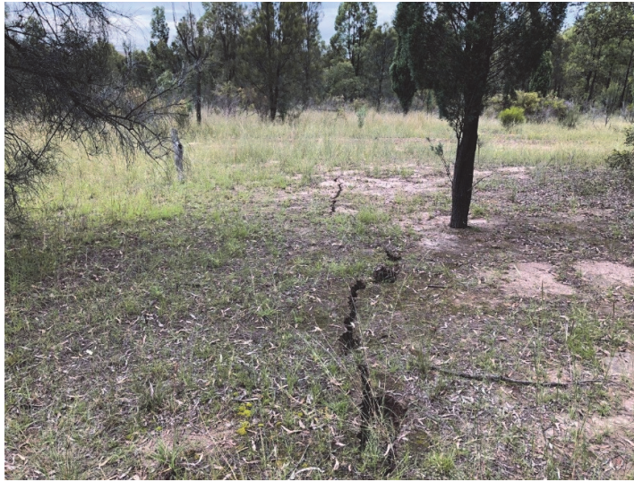
Fig. 4.12 Surface cracking adjacent to the tailgate of WYLW20 (Source: WCPL)
