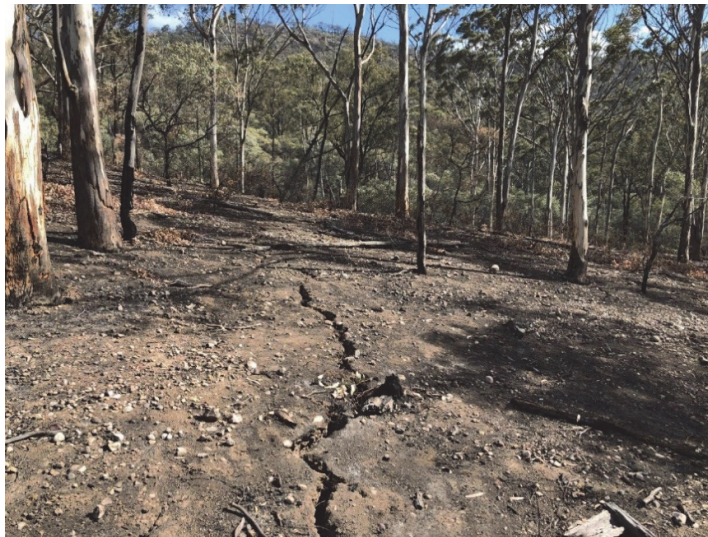
Fig. 4.10 Surface cracking on a steep slope above the south-western end of WYLW18
