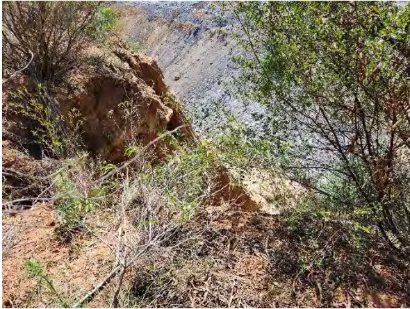
Existing erosion where tributary drops over highwall
