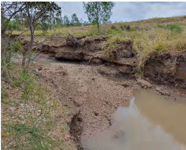
Substantial bank erosion following incision in response to subsidence between LW16 and LW17. Limited riparian vegetation providing poor resistance.
