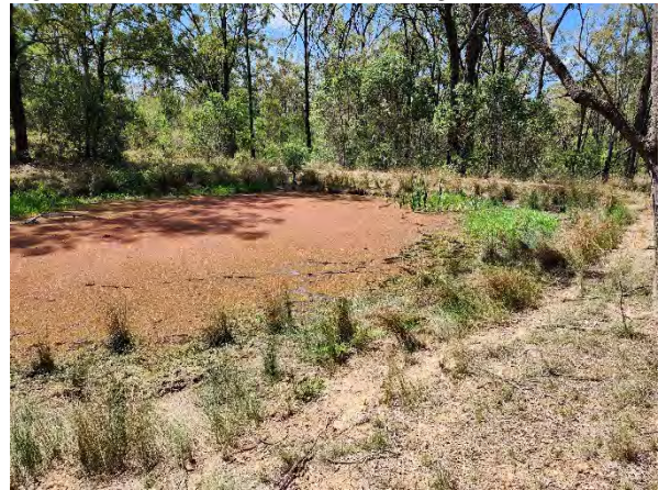
Small dam on LW24-25 pillar that is likely to be destabilised by subsidence
