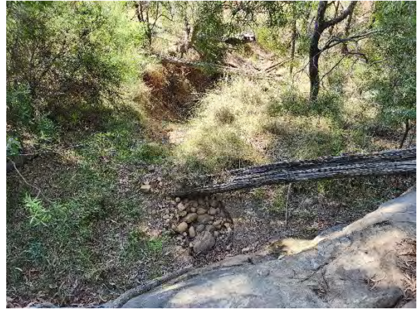
Headcut migration upstream in response to drop over highwall with bedrock control limiting extent
