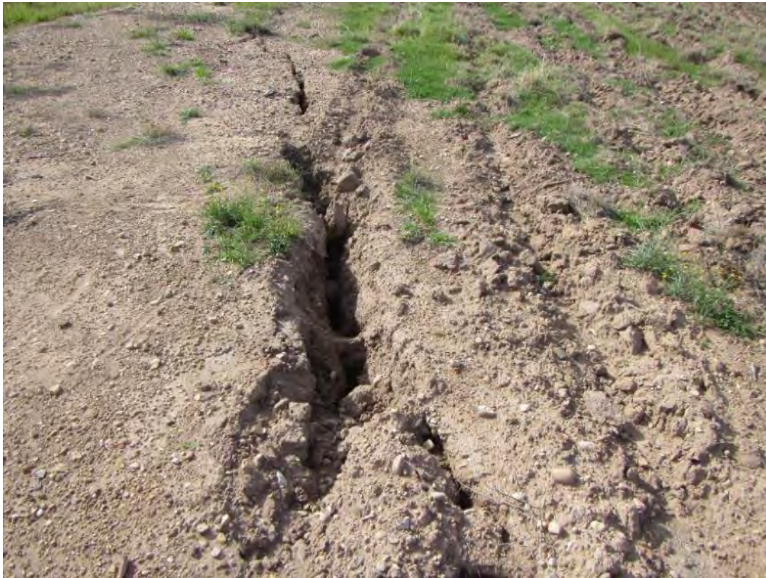
Figure 3-4. Cracking at surface over LW13/14
