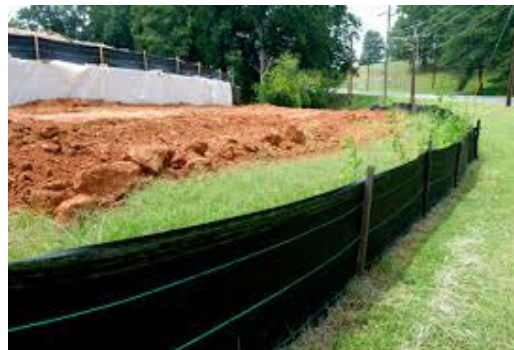
Figure 9: Example of Sediment Fencing
