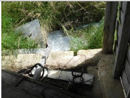
Figure 28: A detail of the banded concrete floor with the timber studs emerging from the edge of the concrete.
