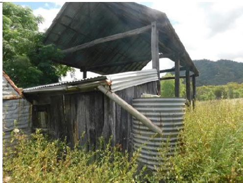
Figure 10: Hayshed looking west across the dwelling.
