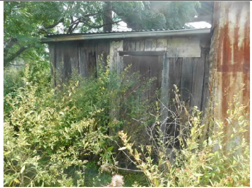
Figure 21: East facade southern half showing the door from the outside.
