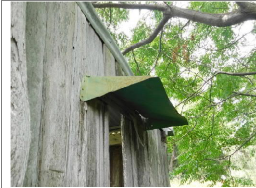
Figure 18: Hood over southern window for weather protection demonstrates occupation.
