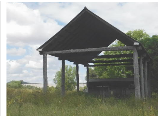
Figure 8: Hayshed looking east with the dwelling at the far end. A simple rural structure of post and beams with a gable roof atop.
