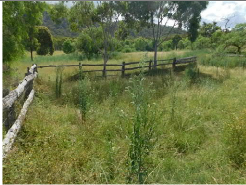
Figure 38: The yards looking northwest. The yards are overgrown and the fence is showing weather damage.
