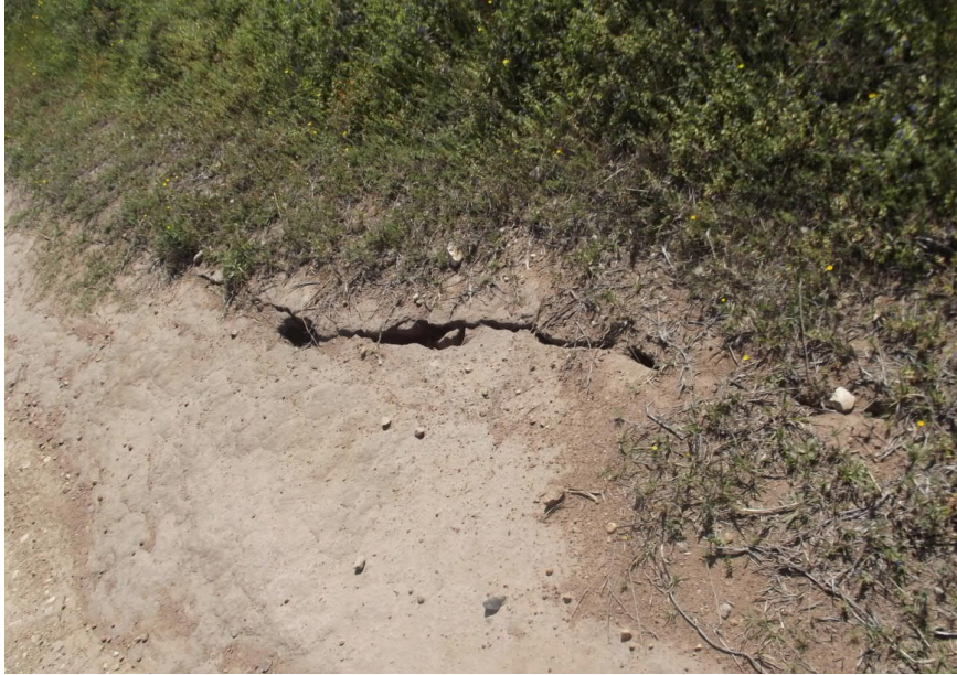
Figure 54: Cracking effect shows the elongated fissure opening into a deep cavity below.
