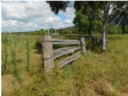
Figure 40: The yards looking southeast. The yards are overgrown and the fence is showing weather damage.
