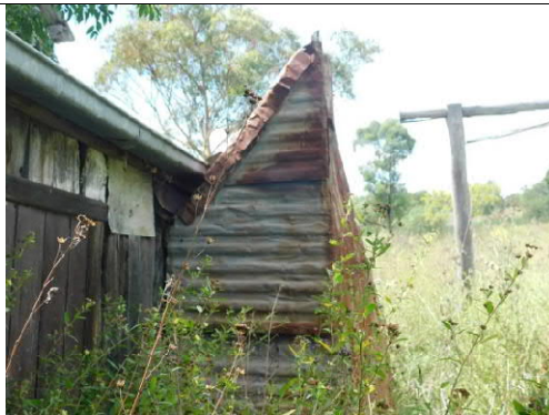
Figure 22: The flue constructed of folded over galvanised iron sheeting
