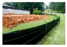
Figure 9: Example of Sediment Fencing
