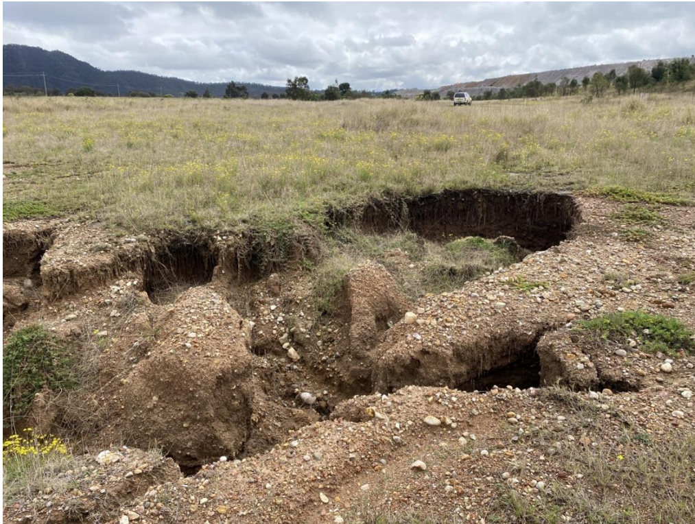
Photograph 18: Gully erosion within the North Wambo Creek Diversion (near site 23R) in 2022
