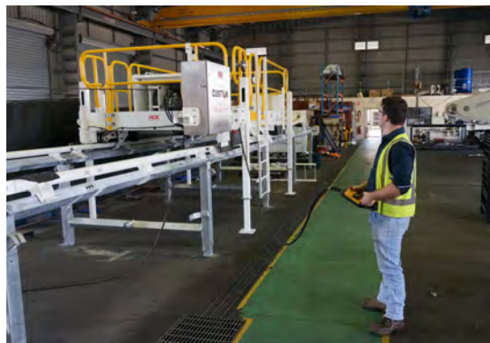
A mobile bolting platform, pictured, enables continuous operation of the conveyor belt and minimal disruption to production at the longwall face.
