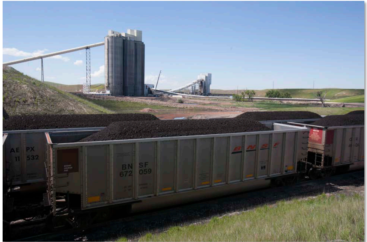
North Antelope Rochelle Mine Loadout Facility
