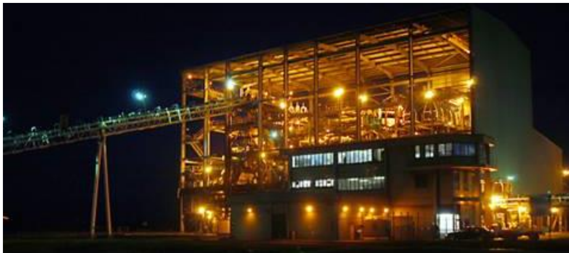
North Goonyella Mine Prep Plant
