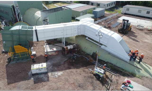
North Goonyella Fan Installation
