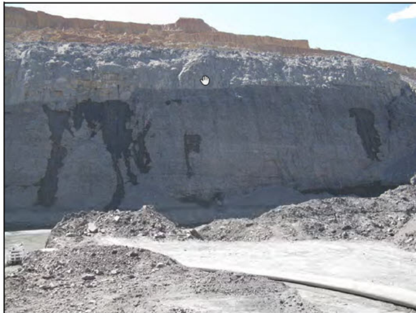
Figure 24. Localised Seepage from fractured Permian Overburden - Coppabella
