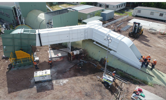
North Goonyella Fan Installation
