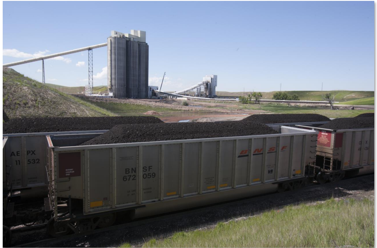
North Antelope Rochelle Mine Loadout Facility
