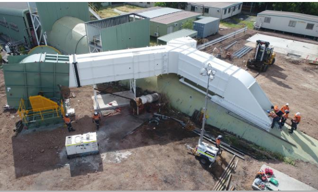
North Goonyella Fan Installation
