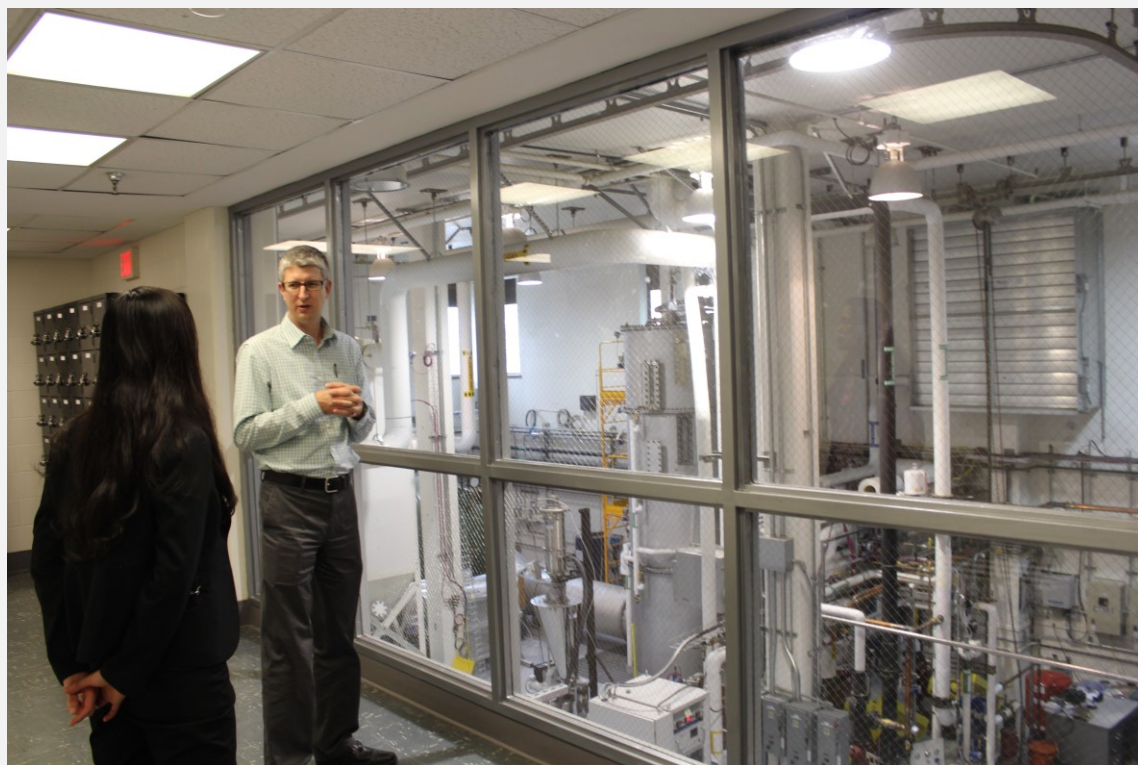
A view overlooking the Advanced Coal & Energy Research Facility at Washington University in St. Louis, where the Consortium for Clean Coal Utilization engages the world's best minds in clean coal research and aims to improve public understanding of coal as a source of energy. Peabody is a founding member of the consortium and has committed $6.5 million since its inception.
