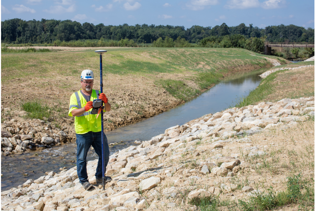
Rich Williams, performing an as-built survey of reconstructed Smith Fork Creek at Somerville Mine.
