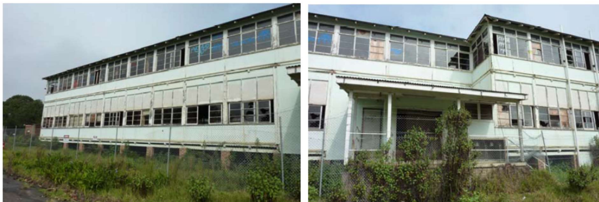
Plates 1 & 2 – Abandoned Hospital Buildings [A01a] {Former Male Wards} (Source: MSEC, 2016)
