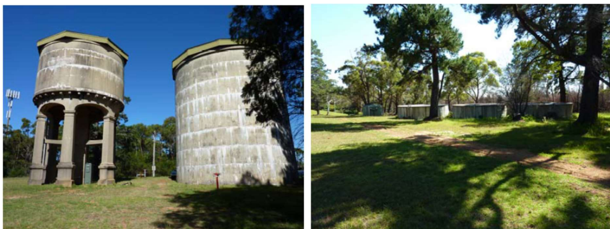
Plates 15 & 16 – Large Water Storage Tanks (Source: MSEC, 2016)
