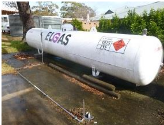
Figure 10 Gas Storage Tank B01t03
