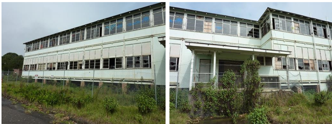
Figure 1 Hospital Building Structure (Ref. A01a)
