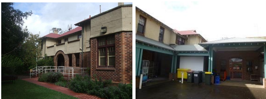
Figure 4 Aged Care Building Structure Ref. B01e
