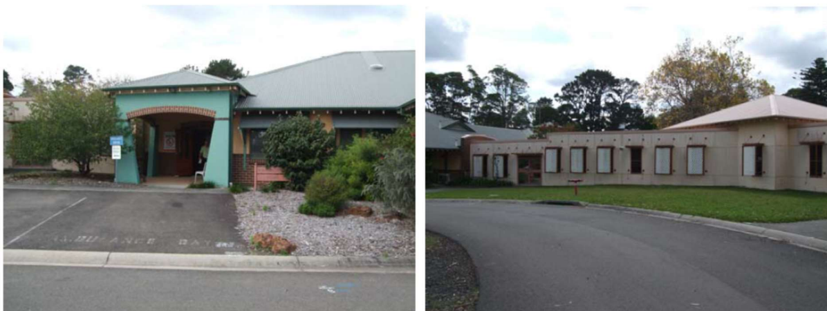
Plates 5 & 6 – Aged Care Building Structures [B01a-B01d] {Administration} (Source: MSEC, 2016)
