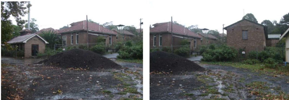
Plates 3 & 4 – Abandoned Hospital Buildings [B03a] {Laundry / Boilerhouse} (Source: MSEC, 2016)
