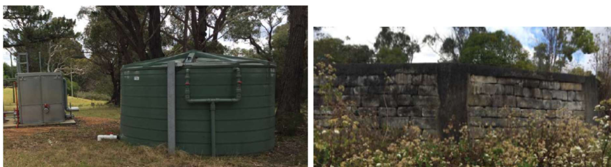
Plates 17 & 18 – Fire Water Tank and Steel Tank Adjacent Pump House, and Trickle Filter Tank (Source: MSEC, 2016)
