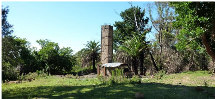
Plate 20 – Kiln (Source: JMA, 2016)
