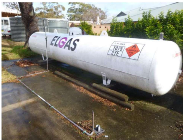
Plate 19 – Gas Storage Tank (Source: MSEC, 2016)
