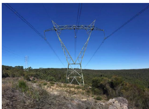
Plate 1 – 330 kV Transmission Tower (Source: MSEC, 2019b)
