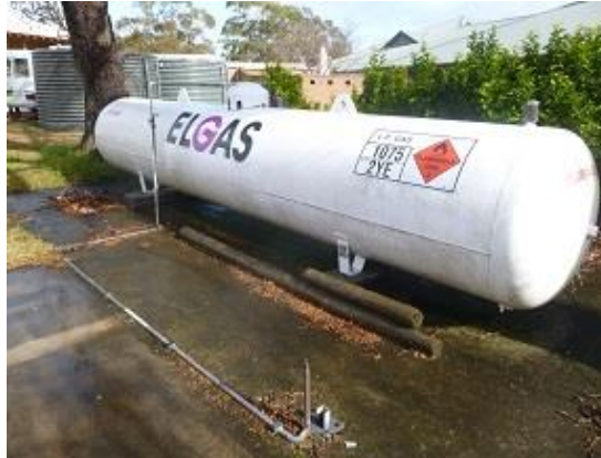
Figure 10 Gas Storage Tank B01t03
