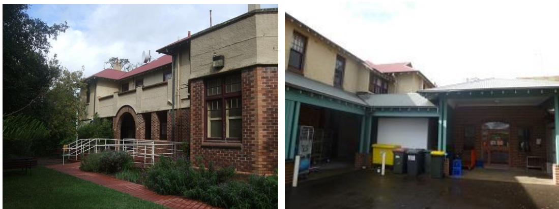
Figure 4 Aged Care Building Structure Ref. B01e
