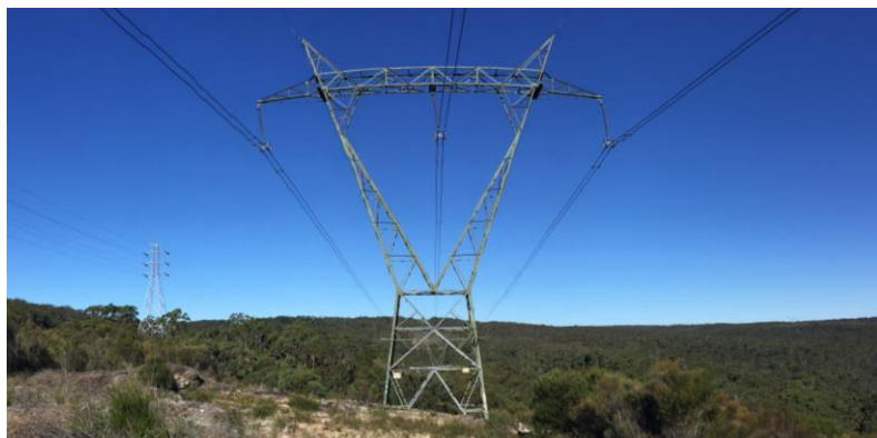
Figure 1 Photograph of a 330 kV Transmission Tower
