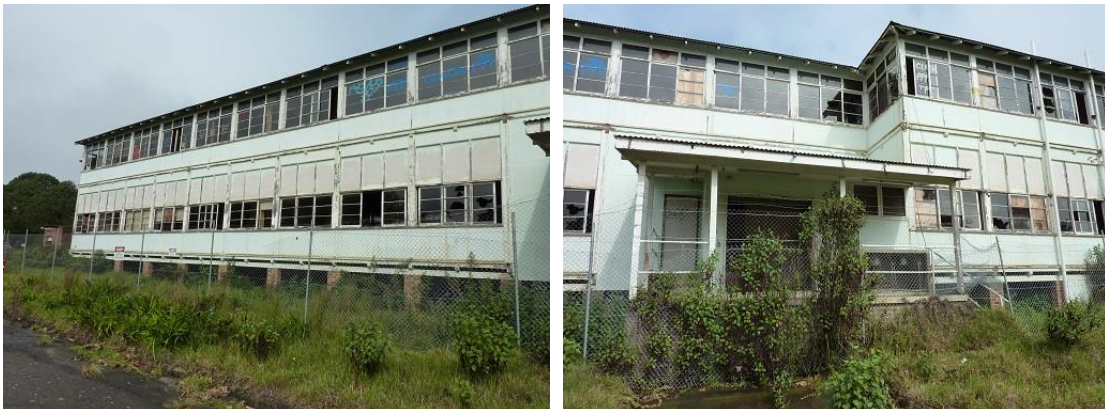
Figure 1 Hospital Building Structure (Ref. A01a)
