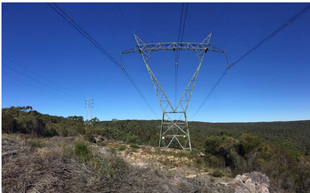
Figure 1 Photograph of a 330 kV Transmission Tower
