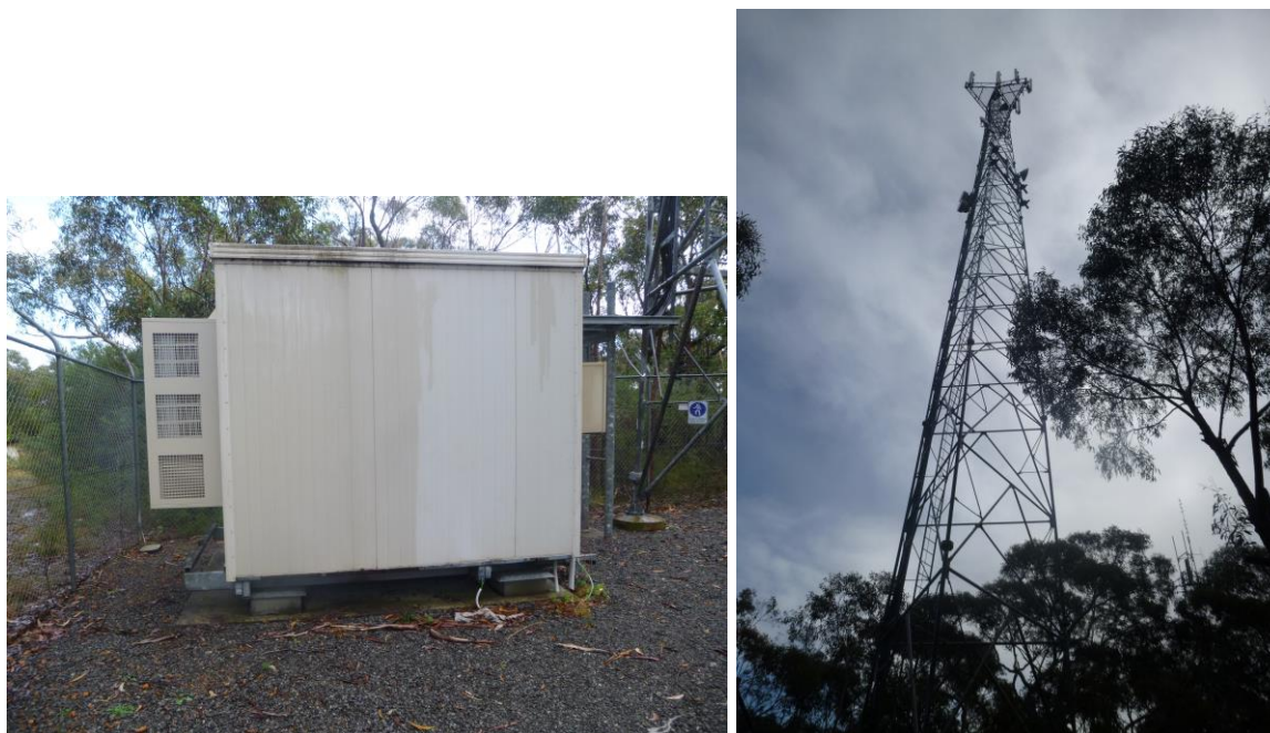
Figure 2 Axicom Telecommunications Tower 2 and Compound
