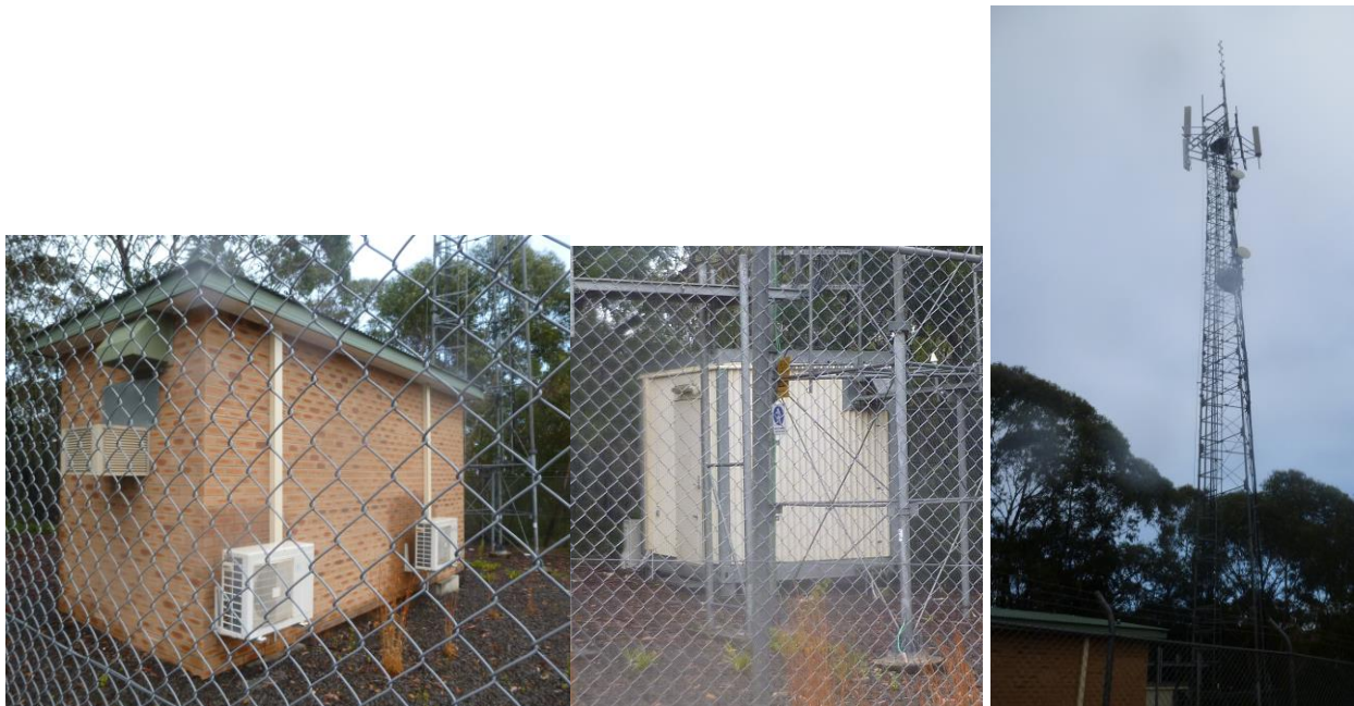
Figure 1 Axicom Telecommunications Tower 1 and Compound
