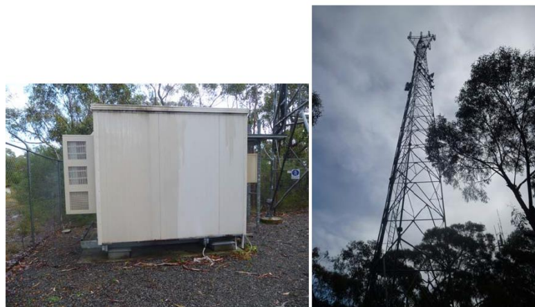
Plates 3 & 4 – Telecommunications Tower 2 and Compound (Source: MSEC, 2016)
