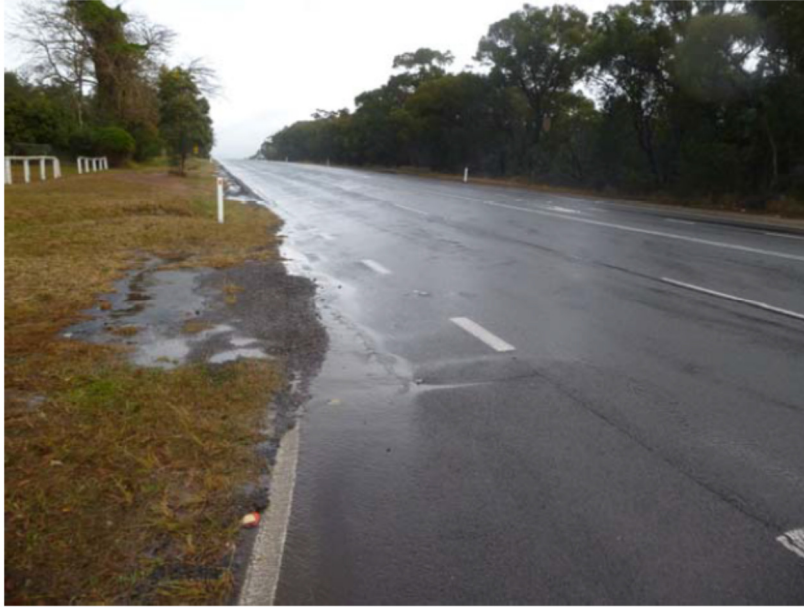
Plate 1 – Old Princes Highway (Source: MSEC, 2016)
