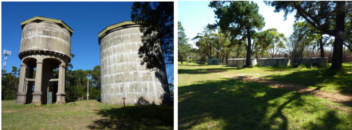
Plates 15 & 16 – Large Water Storage Tanks (Source: MSEC, 2016)
