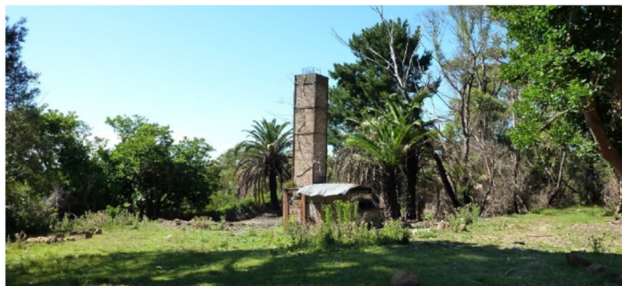
Plate 20 – Kiln (Source: JMA, 2016)
