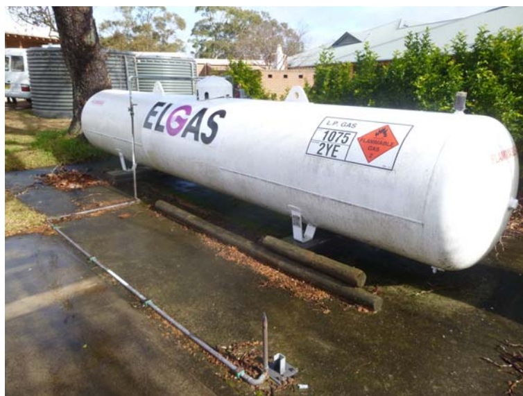
Figure 10 Gas Storage Tanks Refs. B01t03 and B01t04
