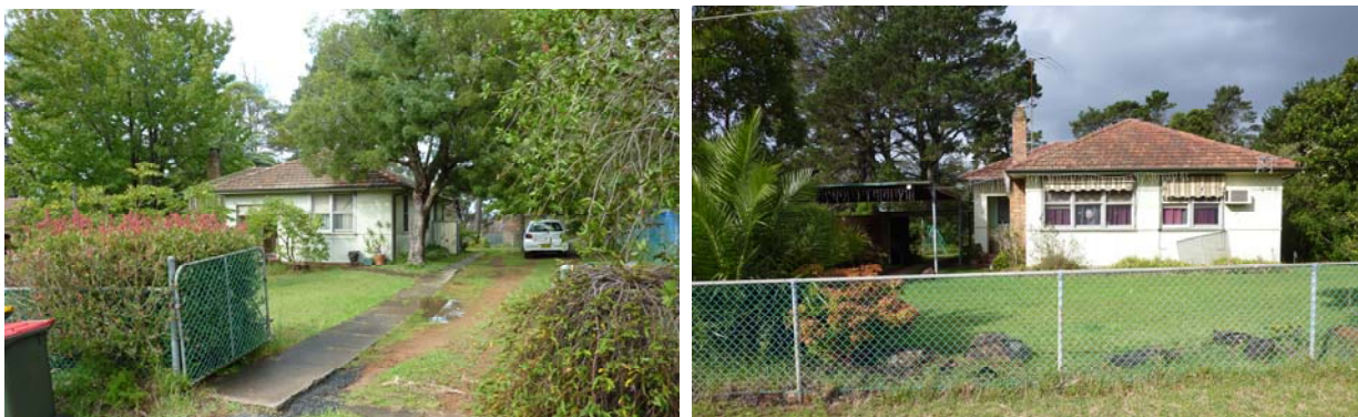
Figure 7 Houses Structure Refs. B06a (left side) and B08a (right side)
