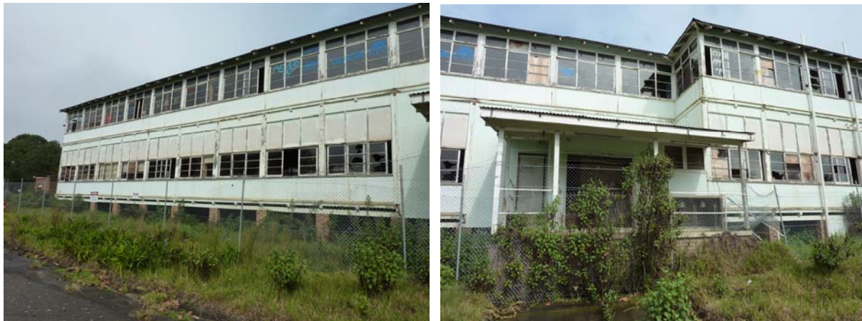
Figure 1 Hospital Building Structure (Ref. A01a)
