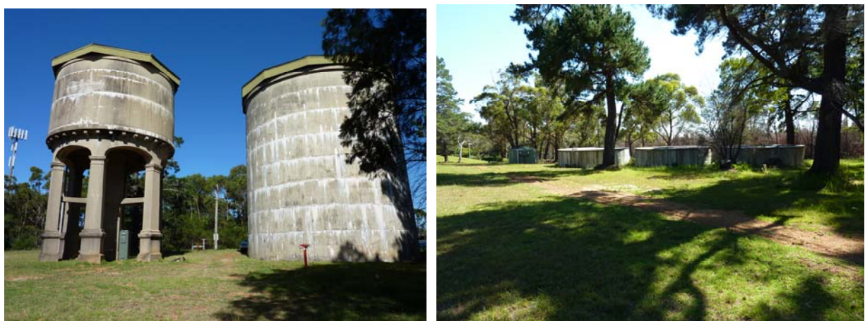
Figure 8 Water Storage Tanks Refs. B14t01 and B14t02 (left side) and Refs. B16t01 to B16t03 (right side)
