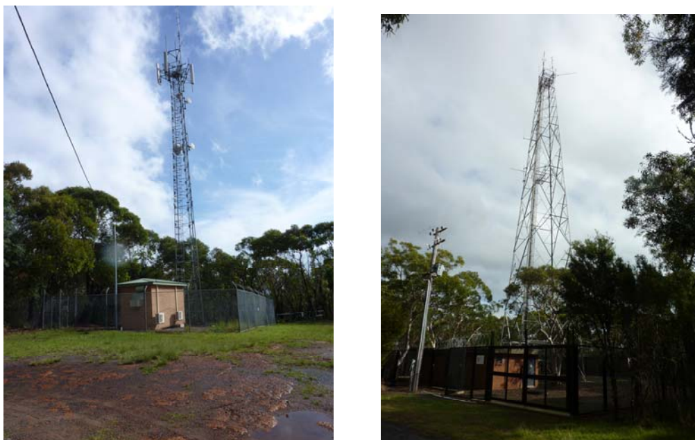
Figure 12 Telecommunications Towers and Compounds Refs. B10a (left side) and B12a (right side)
