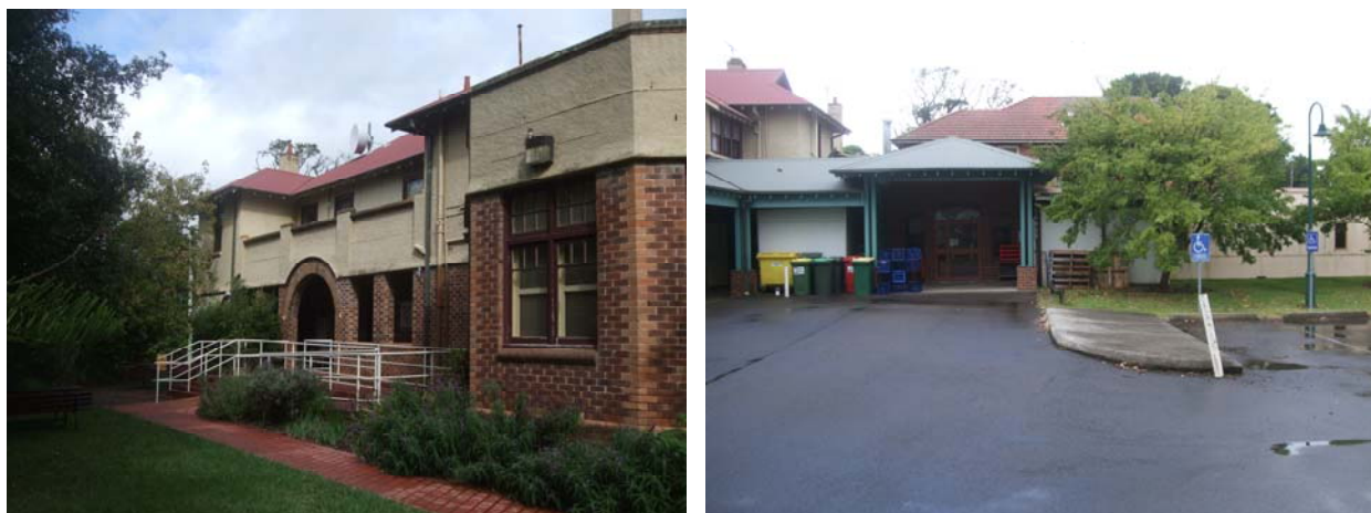
Figure 4 Aged Care Building Structure Ref. B01e
