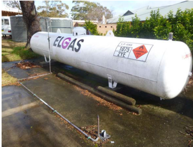
Plate 19 – Gas Storage Tank (Source: MSEC, 2016)
