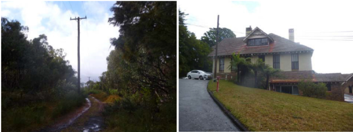
Plates 2 and 3 – Aerial Powerlines (Source: MSEC, 2016)
