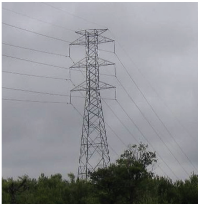
Figure 1 Photograph of a 132 kV Transmission Tower
