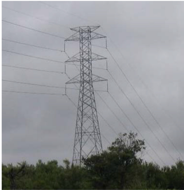
Plate 1 – 132 kV Transmission Tower (Source: MSEC, 2016)
