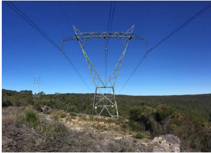
Plate 1 – 330 kV Transmission Tower (Source: MSEC, 2016)
