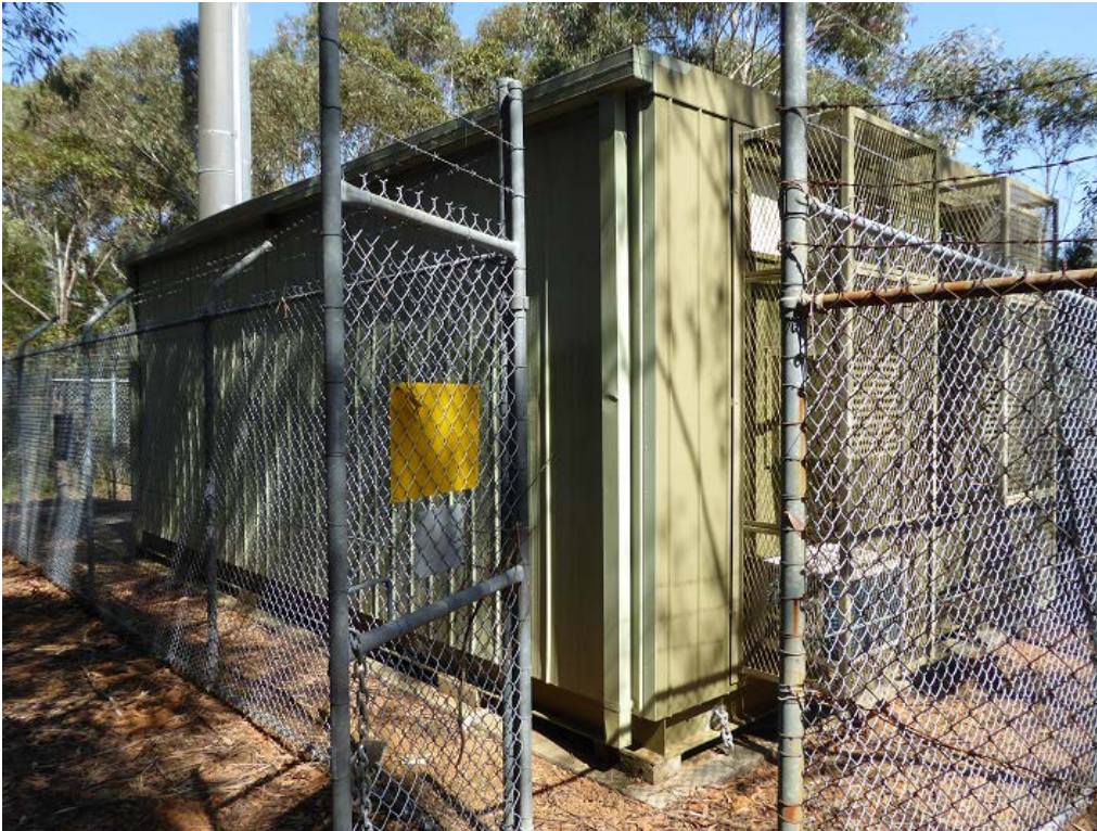
Plate 7: View of Hut at Tower base housing all the transmission equipment for the support of the Mobile Telephone Tower. There is a very heavy battery array at the north end and a check should be maintained that the building is adequately supported at all times
