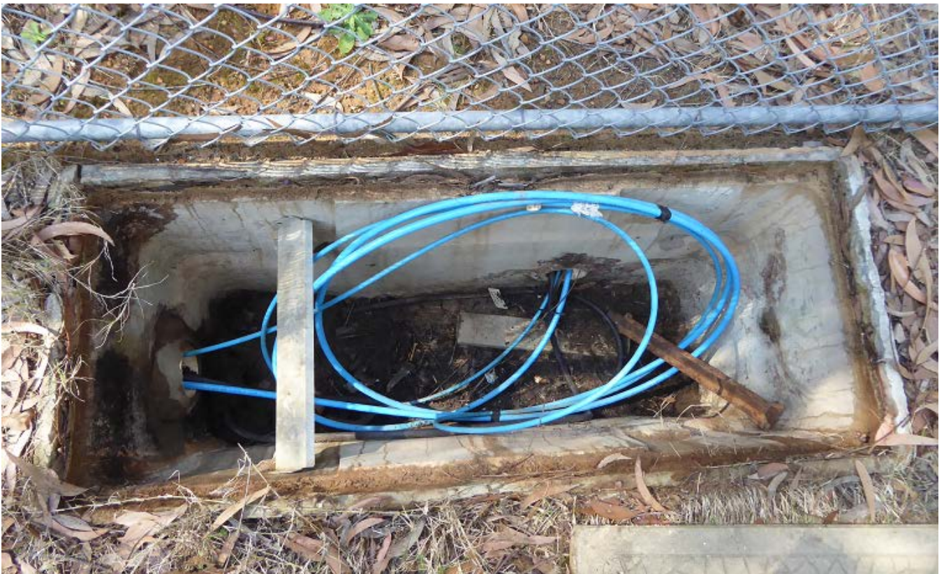
Plate4: Cable entry to Mobile Telephone Tower Hut showing two optical fibre cables into the Hut the larger diameter cable is F ENGA 3005 and the smaller diameter cable is the more vulnerable cable F ENGA 3001.
