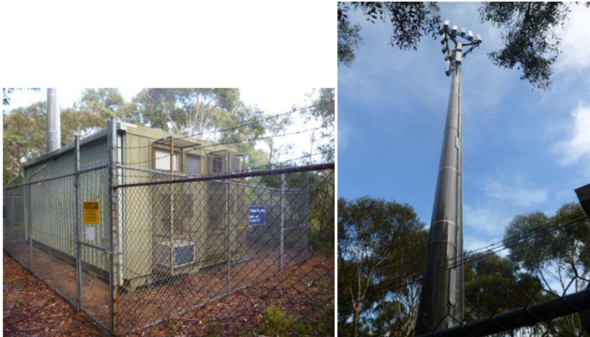
Plates 1 & 2 – Telecommunications Tower and Compound (Source: MSEC, 2016)
