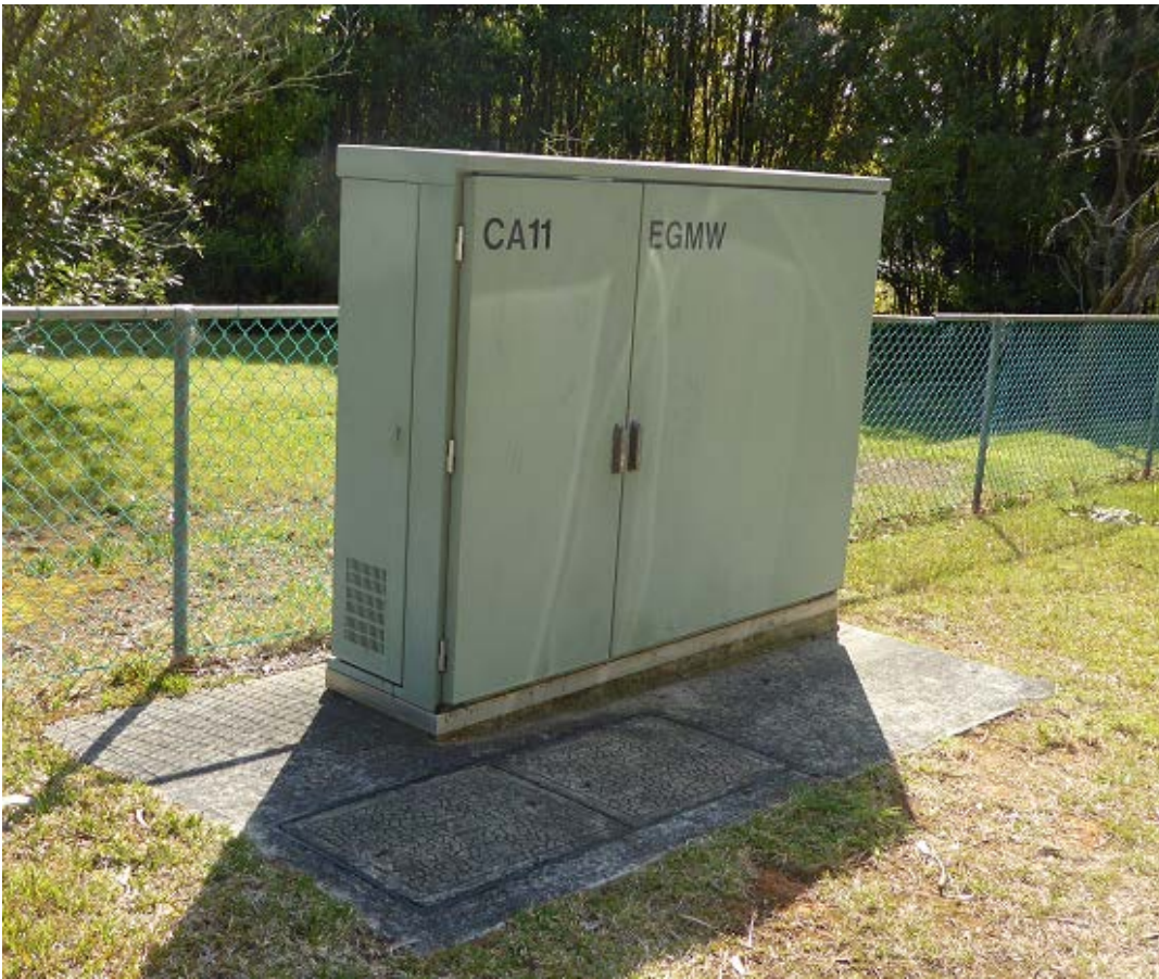
Plate 3: RCM cabinet 'EGMW' located on the access road to the Hospital. Provides copper cable customer services from optical fibre transmission
