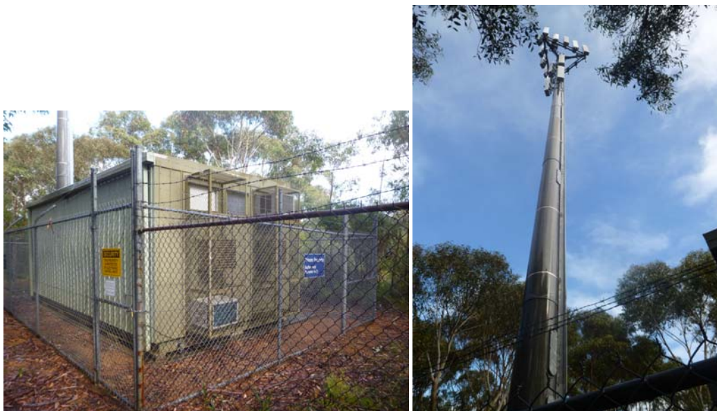
Figure 1 Telecommunications Tower and Compound
