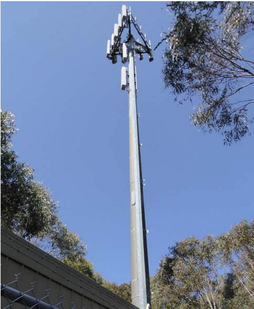
Plate 6: View from western side of 25m steel monopole showing transmission array on north and eastern faces projecting signal towards M1
