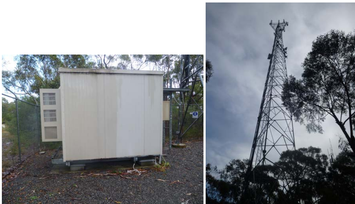
Figure 2 Axicom Telecommunications Tower 2 and Compound
