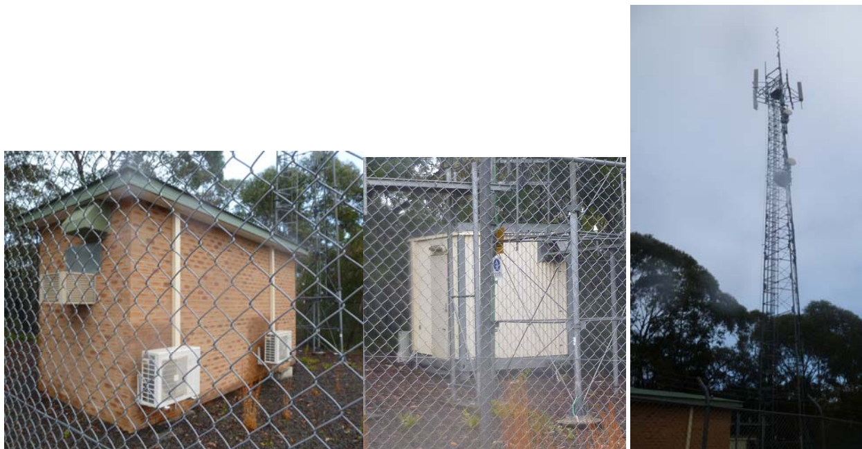
Figure 1 Axicom Telecommunications Tower 1 and Compound
