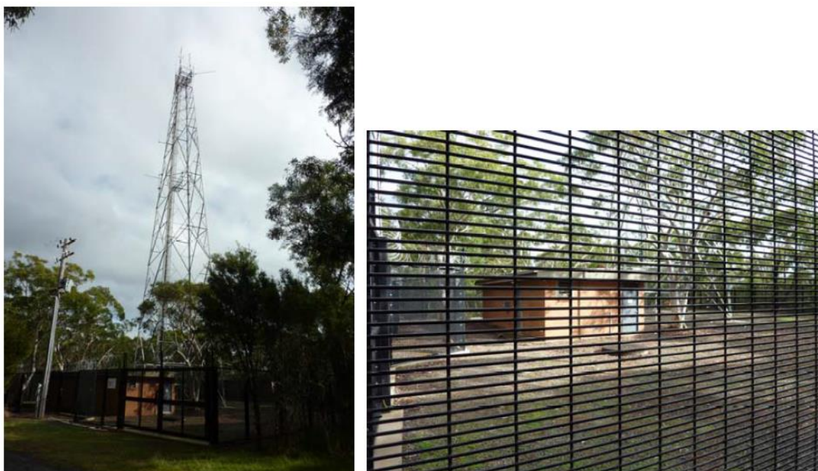
Plates 1 and 2 – Telecommunications Tower and Compound (Source: MSEC, 2016)
