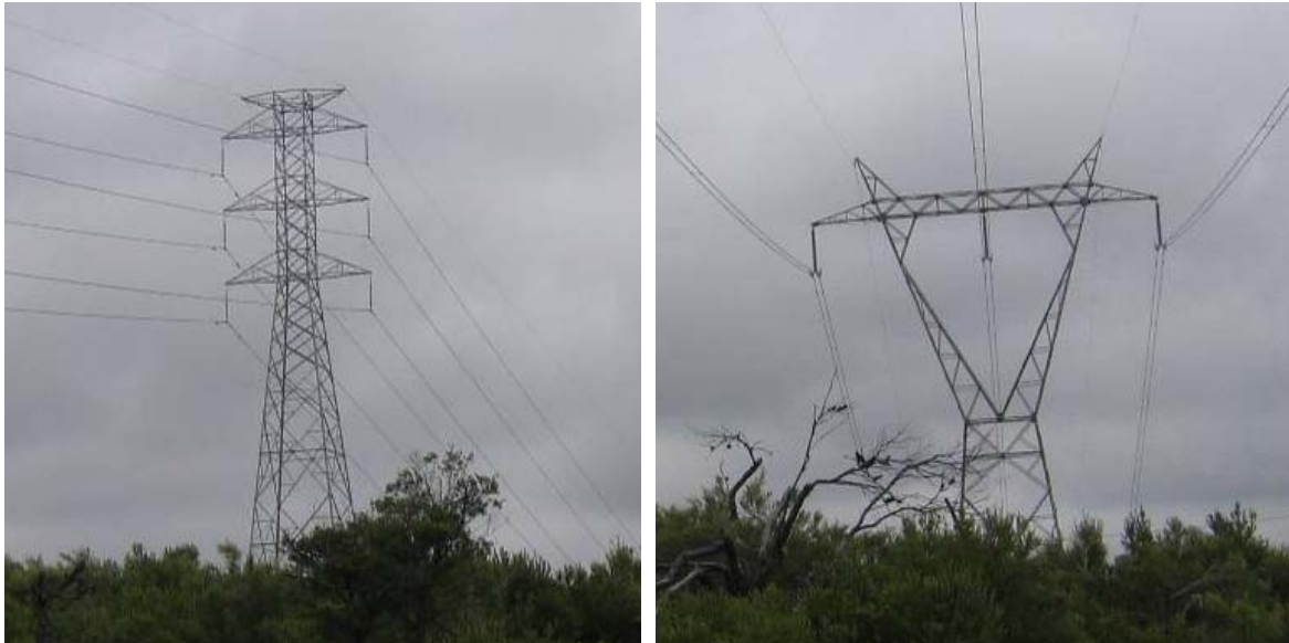
Fig. 6.7 132 kV Transmission Tower (left side) and 330 kV Transmission Tower (right side)
