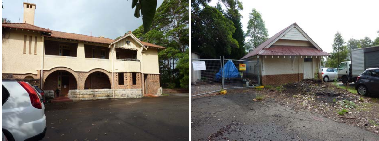
Fig. 11.6 House Structure Ref. A09a (left side) and A09b (right side)
