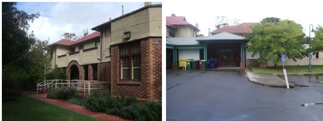
Fig. 11.4 Aged Care Building Structure Ref. B01e
