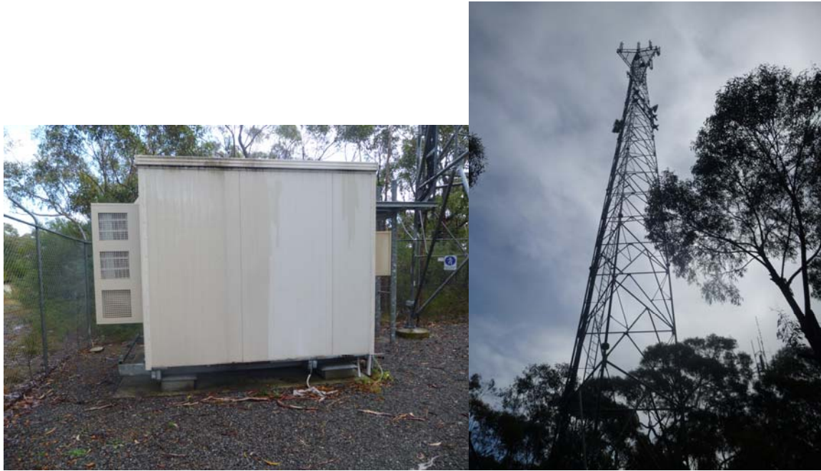
Fig. 6.12 Telecommunications Tower and Compound owned by Axicom
