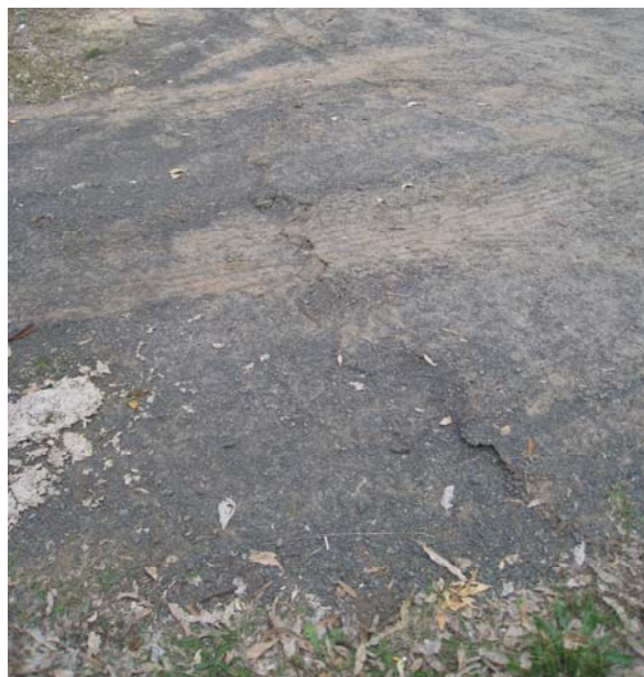
Fig. 4.14 Surface Compression Buckling Observed in a Pavement
