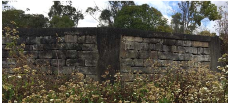
Fig. 11.11 Trickle Filter Tank B15t01
