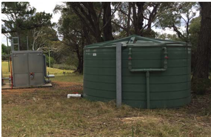
Fig. 11.9 Water Storage Tanks Refs. B17t01 (poly tank) and B18t01 (steel tank)
