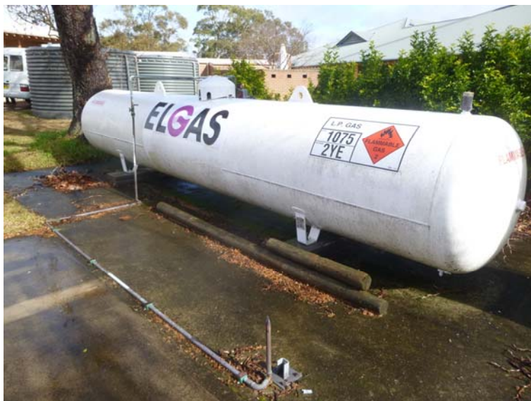
Fig. 11.10 Gas Storage Tank B01t03
