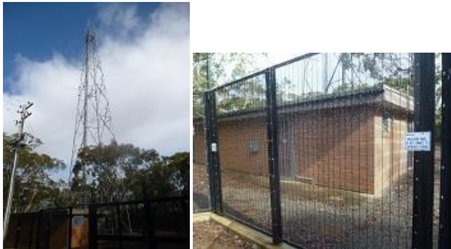
Fig. 6.8 Telecommunications Tower and Compound owned by Sydney Trains
