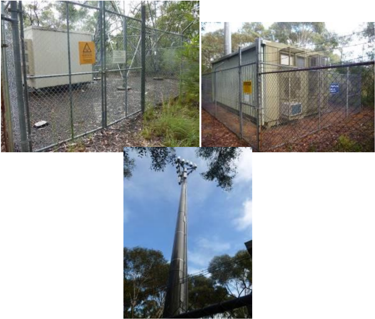
Fig. 6.7 Telecommunications Tower and Compound owned by Telstra
