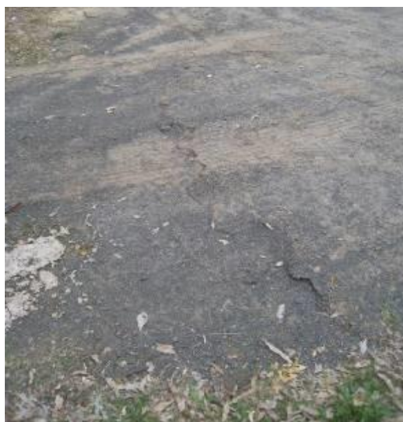
Fig. 4.14 Surface Compression Buckling Observed in a Pavement
