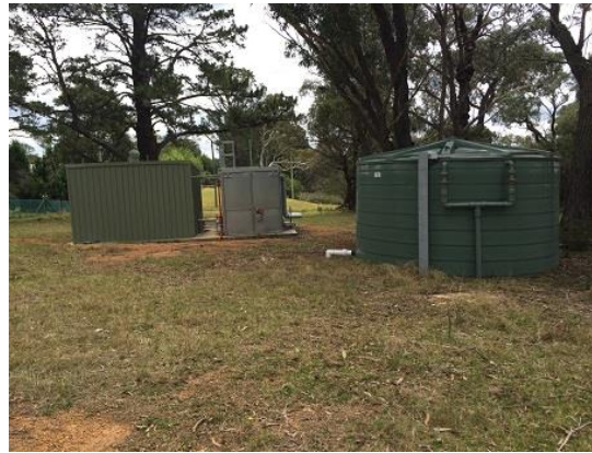
Fig. 11.9 Water Storage Tanks Refs. B17t01 (poly tank) and B18t01 (steel tank)
