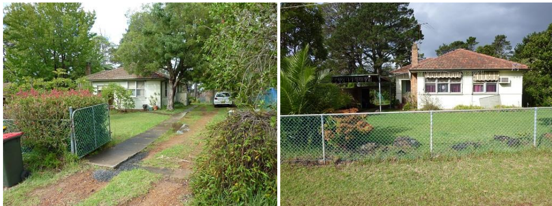
Fig. 11.7 Houses Structure Refs. B06a (left side) and B08a (right side)
