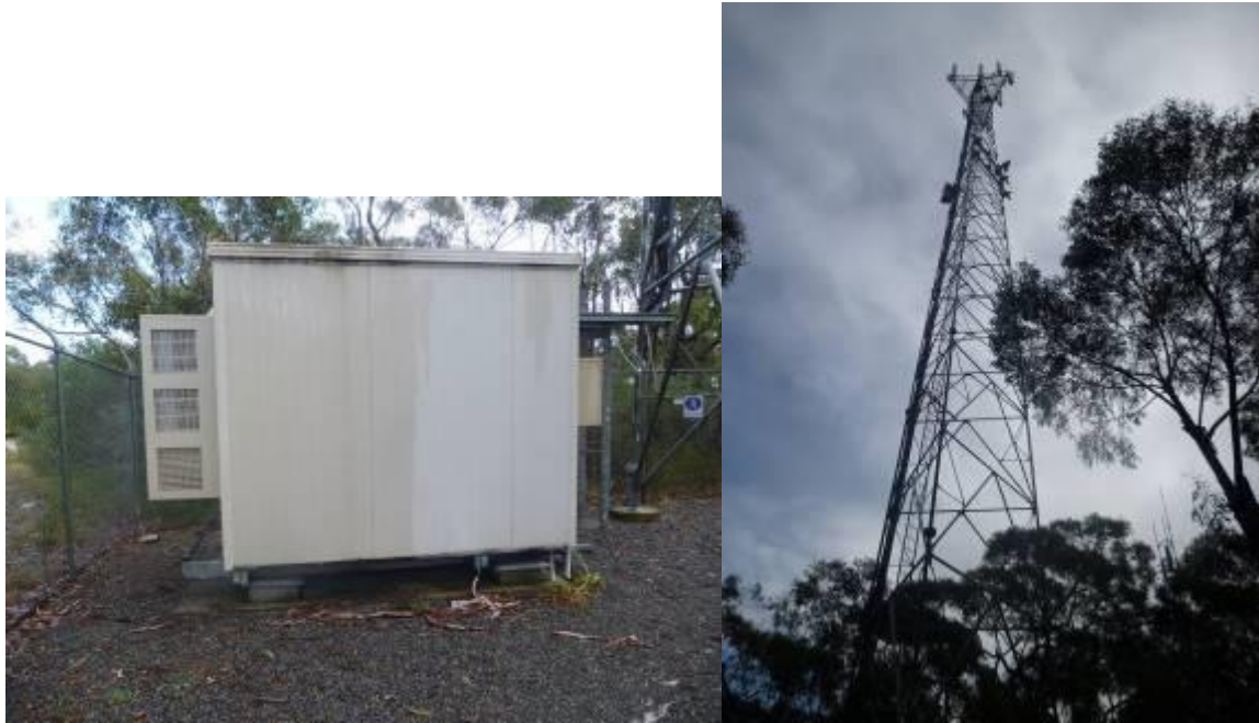
Fig. 6.9 Telecommunications Tower and Compound owned by Axicom
