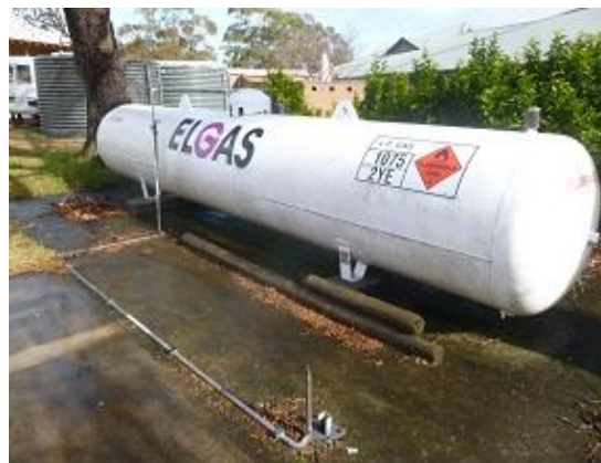
Fig. 11.10 Gas Storage Tank B01t03
