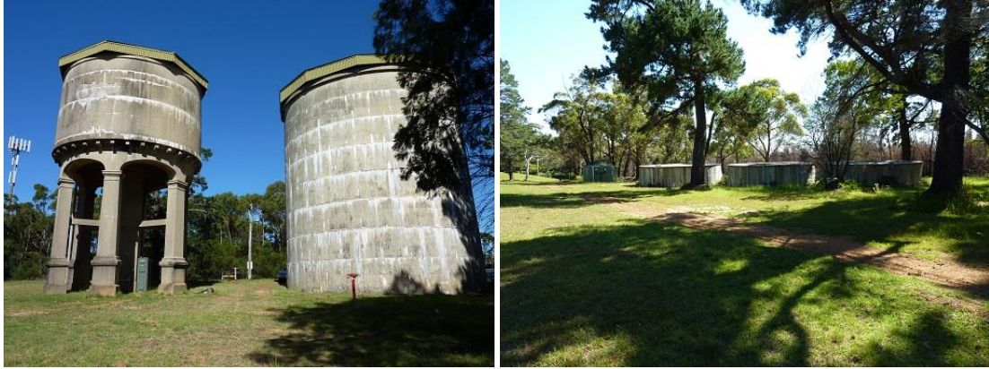
Fig. 11.8 Water Storage Tanks Refs. B14t01 and B14t02 (left side) and Refs. B16t01 to B16t03 (right side)
