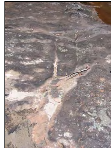
M-4 Joints in Rockbar M
