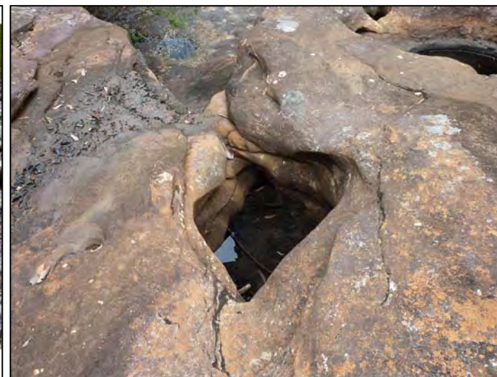
TB145-3 Pothole in overhang
