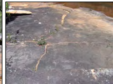
G1-14 Crack perpendicular to joint
