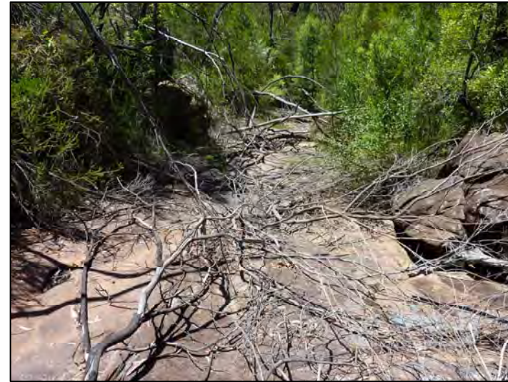
TB040-2 Rockbar looking Downstream
