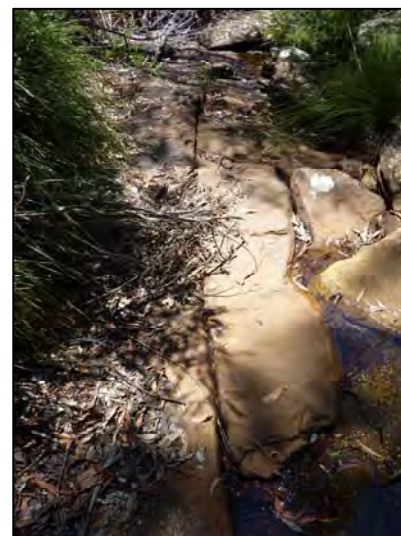
TA23-3 Joint downstream of Pool TA-I
