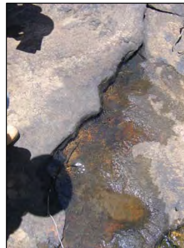
O4-6 Flow emerging at upstream end of Rockbar O4
