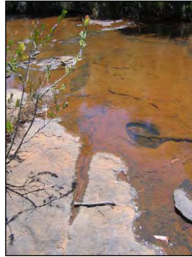
N-4 Joints in rockbar N
