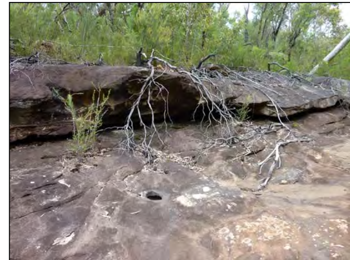
TB142-4 Overhang along southern bank Upstream of Pool TB-AG
