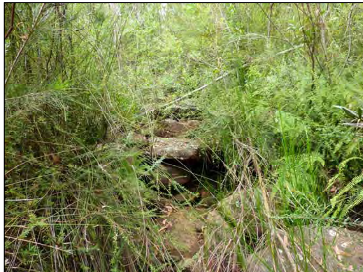
TB151-1 Upstream of Pool TB-AJ looking Upstream
