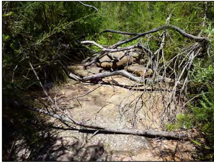
TB047-4 Rockbar looking Downstream
