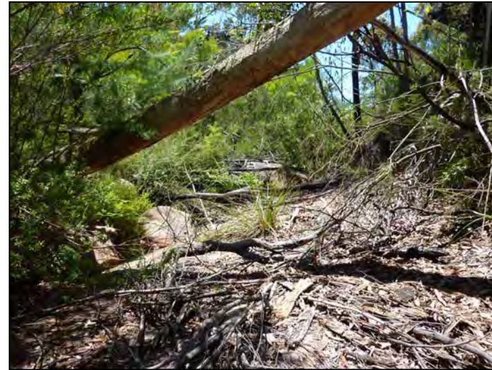
TB037-2 Rockbar looking Downstream
