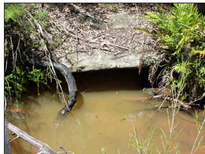
TB022-3 Upstream end of Pool TB-B looking to overhang on eastern bank
