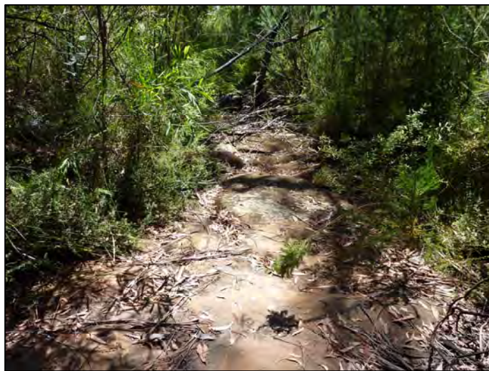
TB048-2 Rockbar looking Downstream
