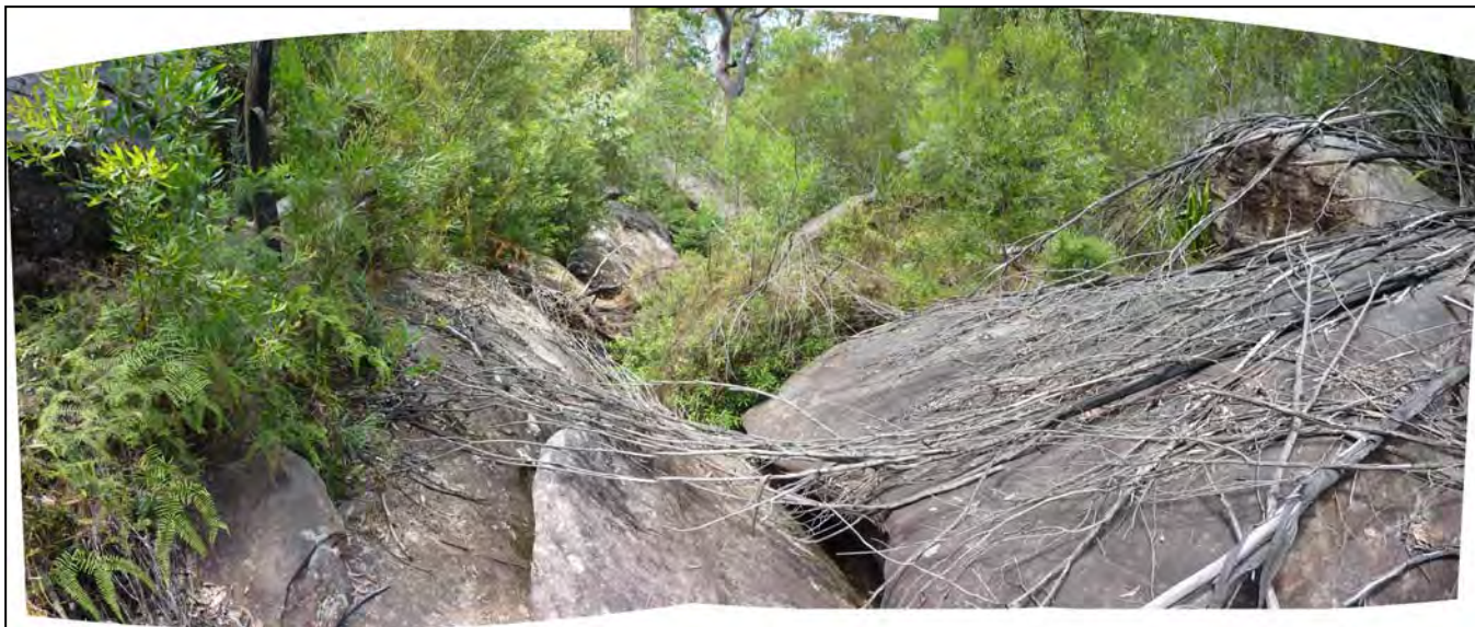
TB078-2 Large detached blocks looking Downstream
