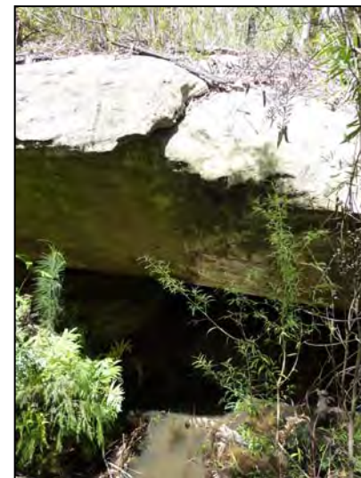
TB100-4 Near Downstream end of Pool TB-M looking toward southern bank
