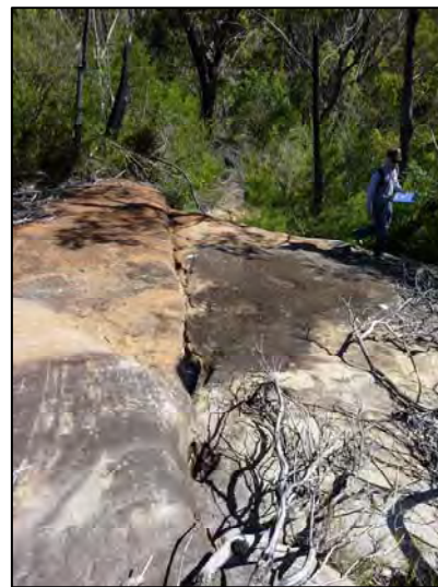
TB069-6 Joint with water
