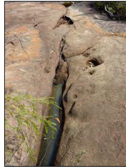
TB120-3 Joint with water
