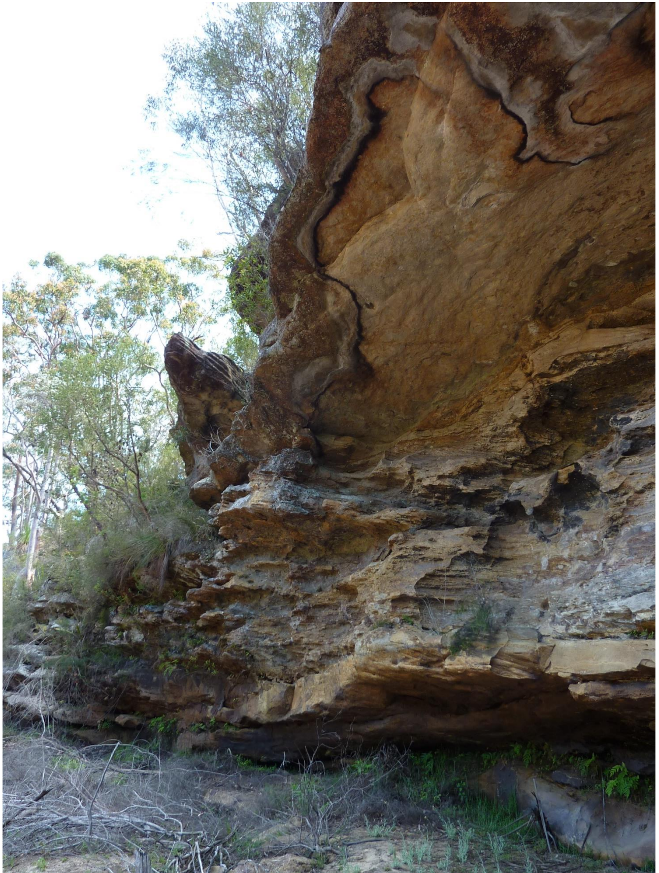
Photo C17-05 View Looking Downstream
