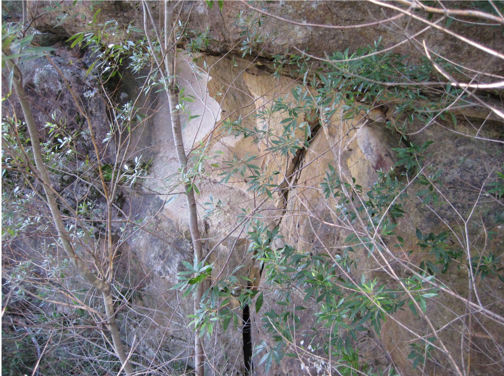
Photo C15-03 Eastern End – Existing Fracture in Rock
