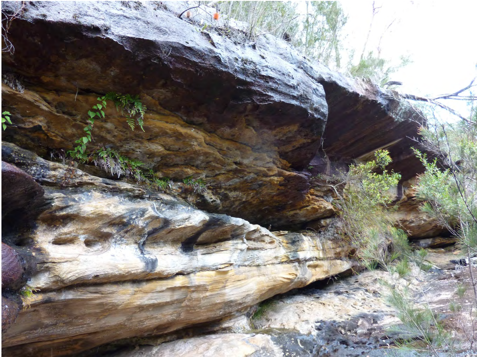
Photo C16-06 View Looking Upstream
