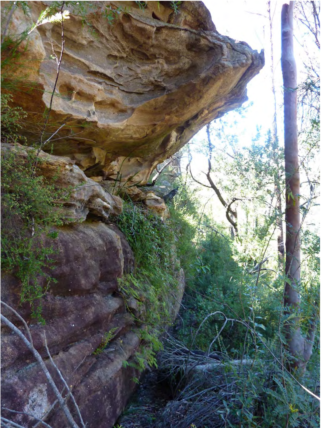
Photo C4-03 Overhang, height ~6m, depth ~3m
