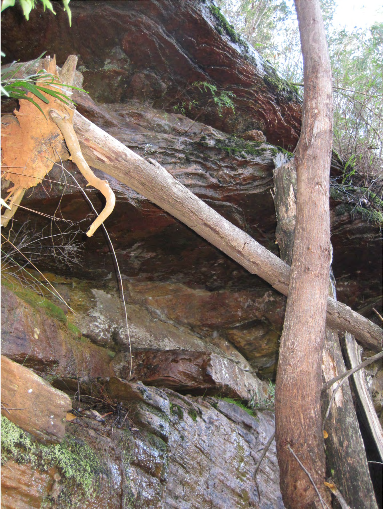
Photo C15-06 Western End Looking Downstream
