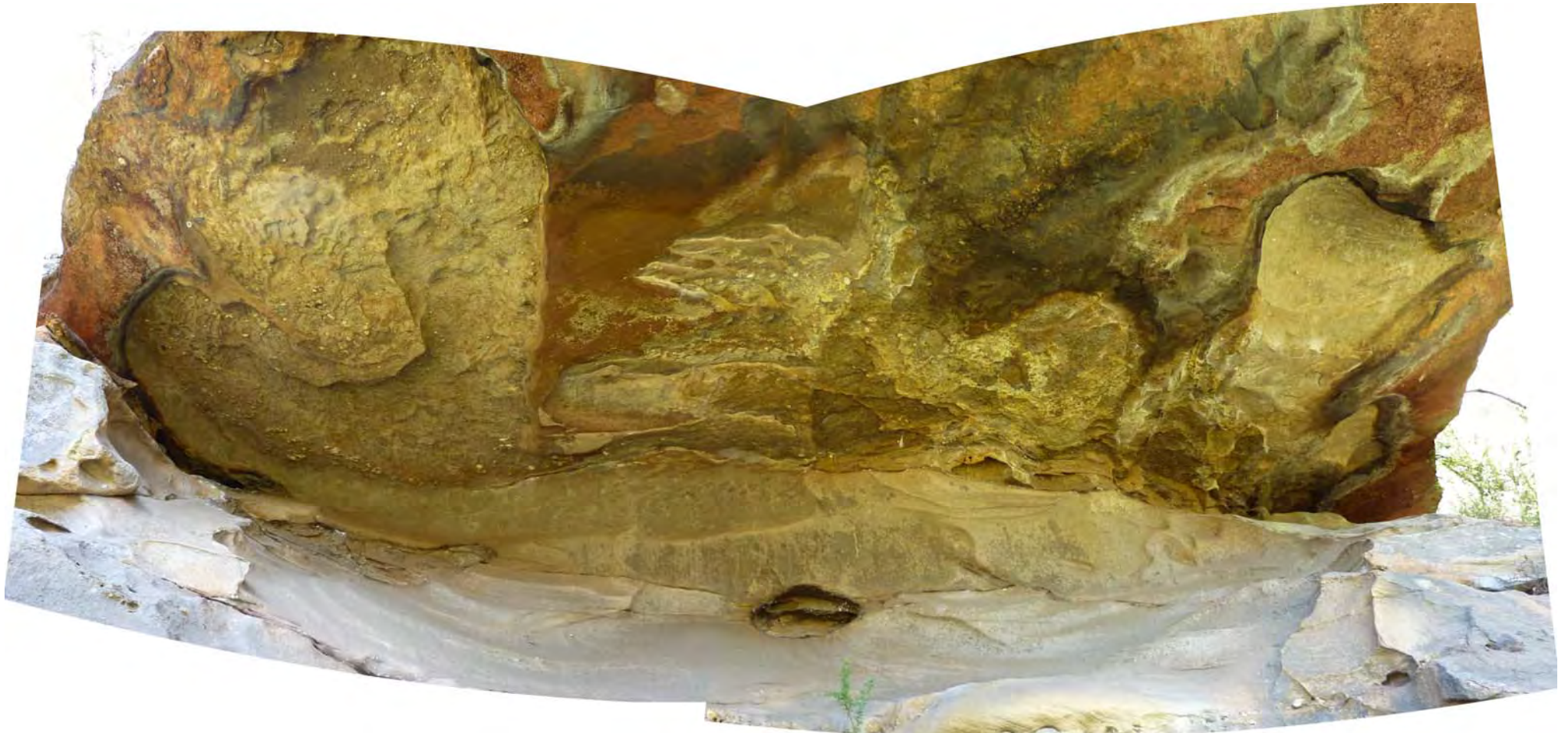
Photo C2-04 Underside of overhang, height ~4m, depth ~3.5m
