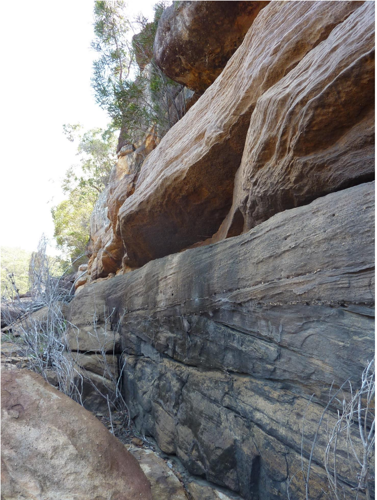
Photo C13-04 South End Looking Downstream
