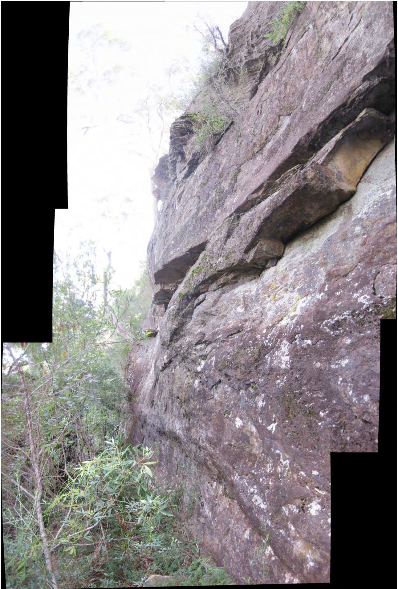
Photo C15-16 View Looking Upstream
