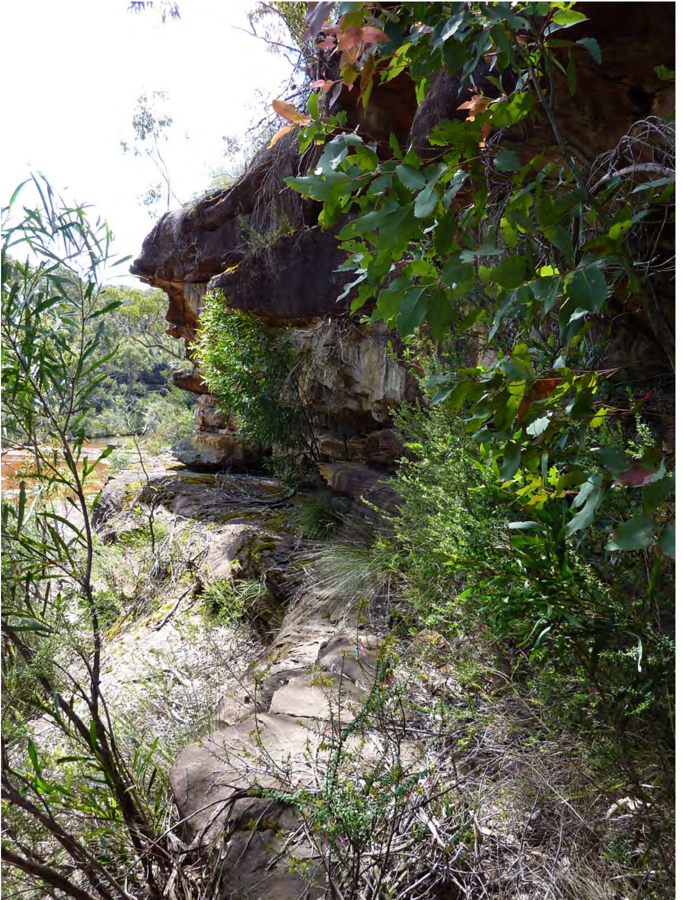
Photo C1-17 Southern end of cliff/Northern end of large overhang
