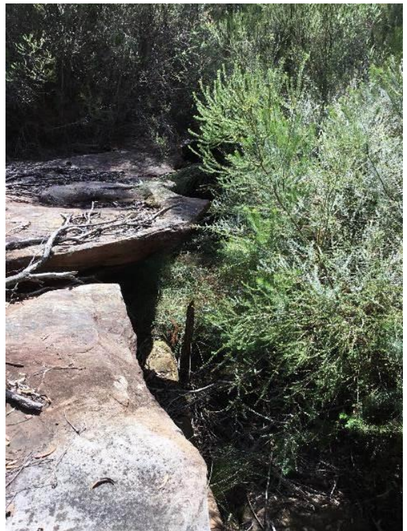
Photo F5 (Downstream)
