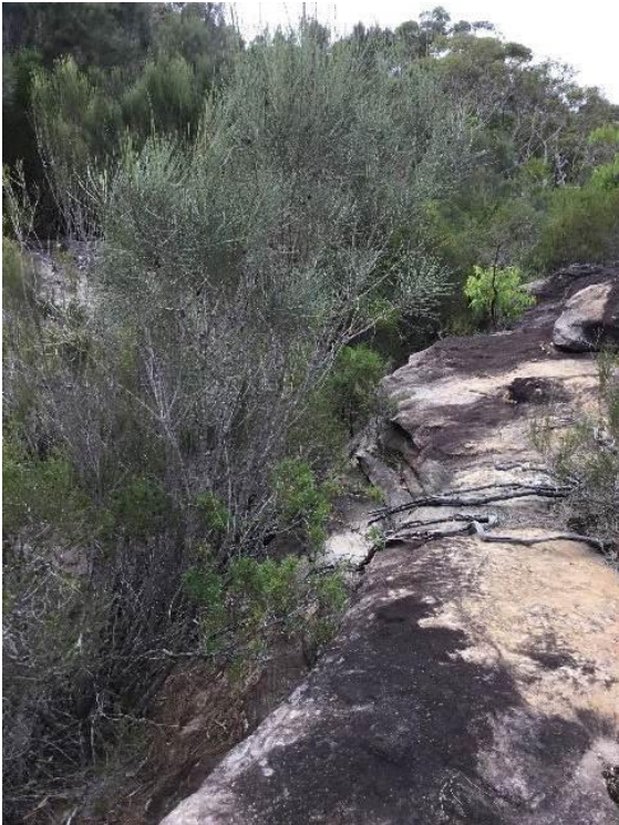
Photo P6 (Downstream)
